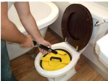
A common occurrence during flooding is back flow through sewage and drainage systems which have been overloaded by floodwater. Even if you have protected your house and managed to prevent floodwater from entering, raw sewage may still flow out of toilets. Toilet covers are available which create an airtight seal in the toilet bowl.
