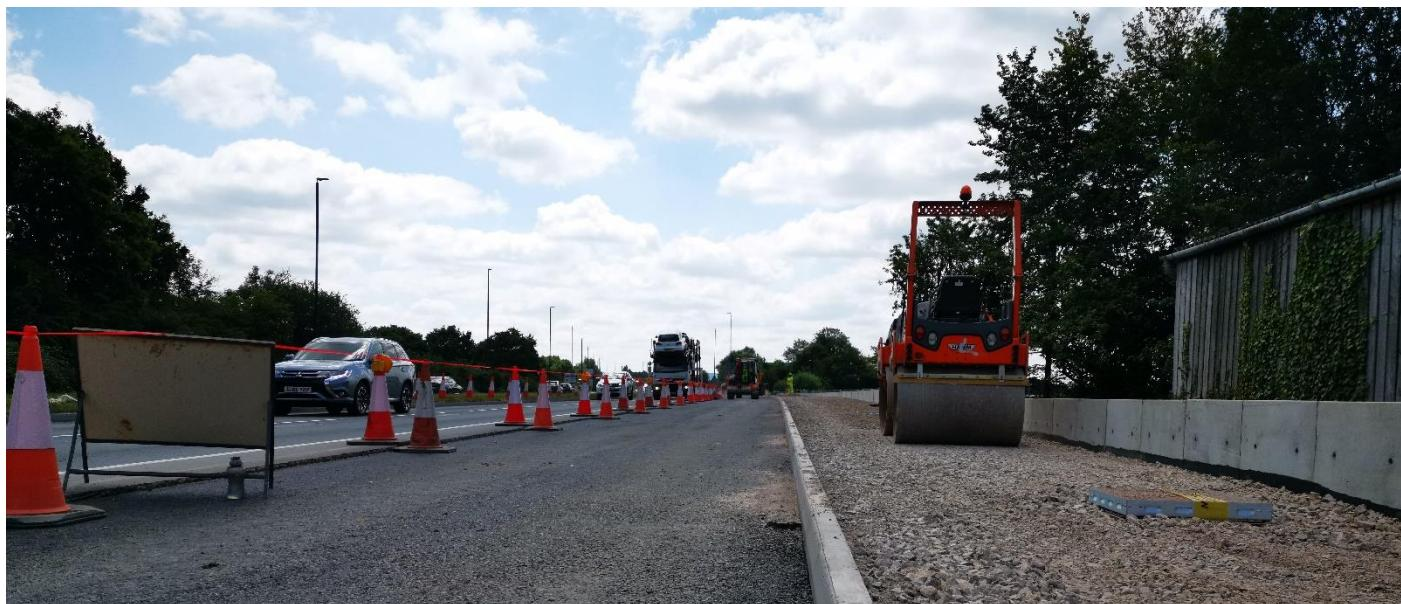
Works have continued in the verge between the A38 approach to Cross Keys Roundabout from Whitminster/Stroud and the A38 towards Gloucester from Cross Keys Roundabout, with drainage being installed and construction of the new widened carriageway started, with the barriers remaining in place for crew safety.
