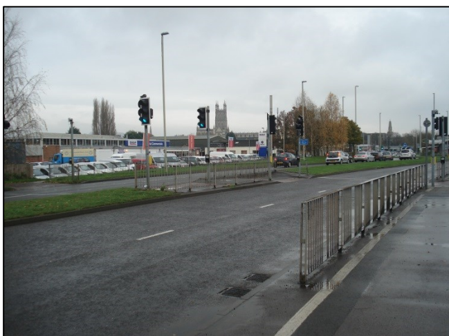
Expectations for strategic network condition are for a higher standard with no running lane defects and a smoother ride quality
