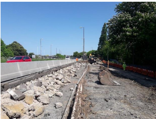
Site clearance towards Whittington Road
