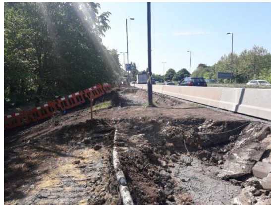
Site Clearance towards Arle Court
