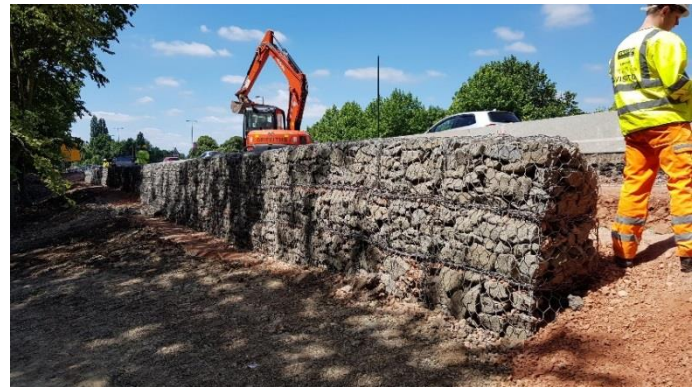
The gabion wall: a structure to support the new road
