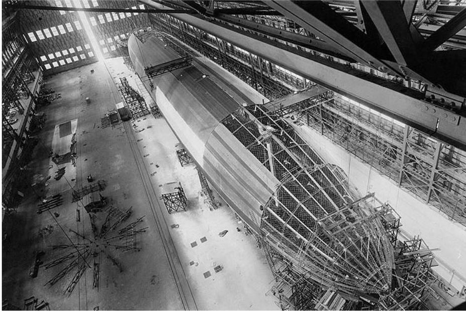
*An American Navy airship under construction, showing the framework.*
