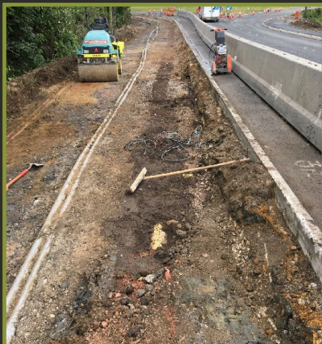
Excavation to expose existing service ducts on the westbound carriageway
