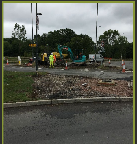
Construction work has commenced to install splitter islands on Grove Lane
