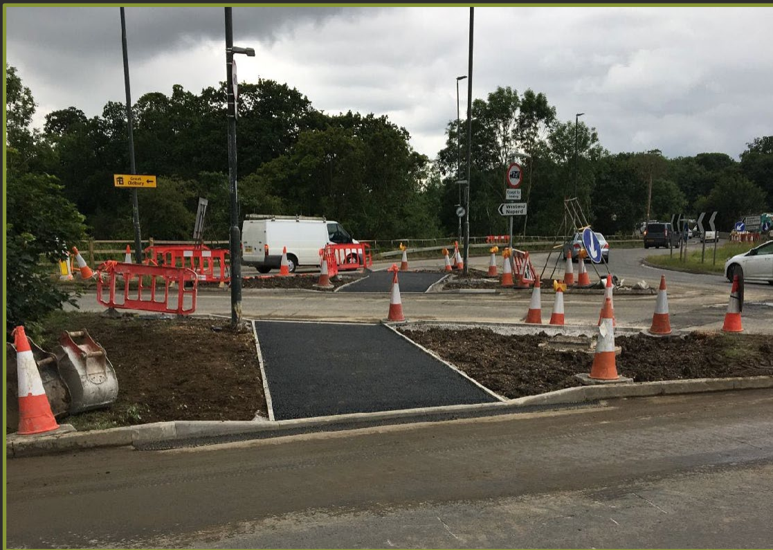
Ducts have been installed and footpaths formed on the Splitter Islands at Grove Lane.
