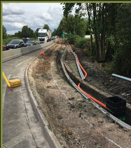
Service ducts have been moved to enable construction of the new road on the westbound approach
