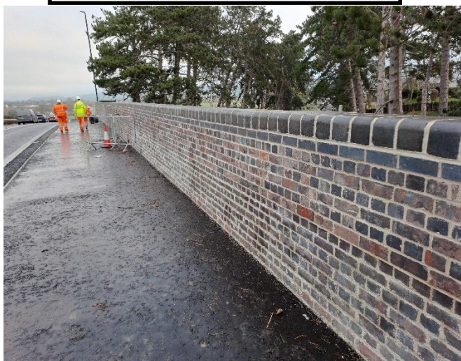
GWSR Bridge – brickwork and repointing completed
