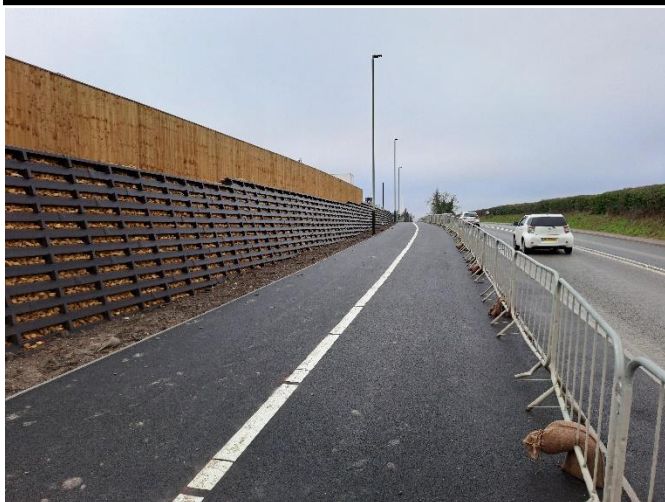
Cheltenham Racecourse Roundabout to GWSR bridge – Cribblock retaining wall, cycleway surfacing and delineator strips installed.
