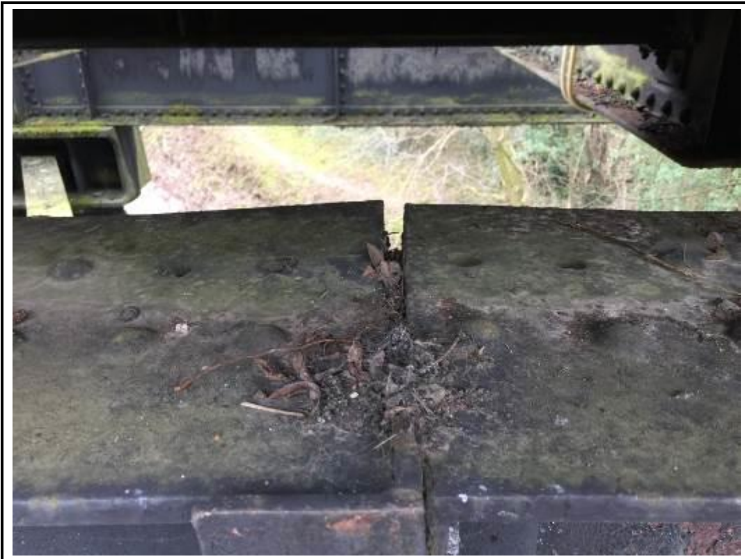
Photo 8. View of distortion and missing rivets, top flange, MGE joins.
