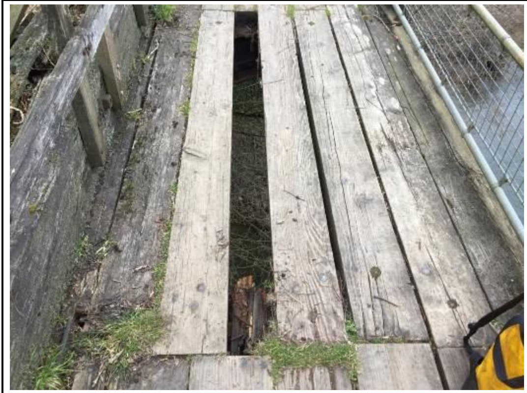
Photo 29. View of missing walkway timber at centre.
