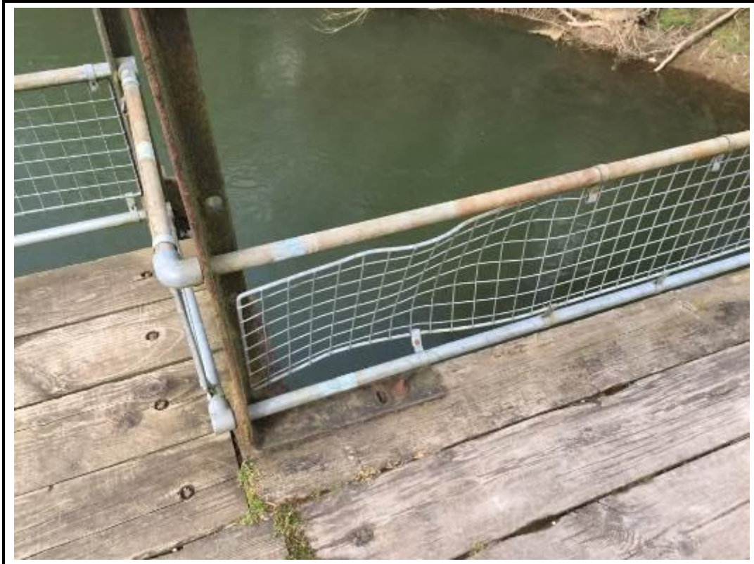
Photo 57. View of deformed galvanised mesh to downside handrail.
