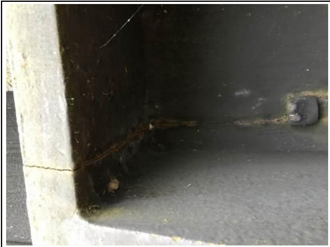
Photo 48. View of fracture through pier 3 downside box.
