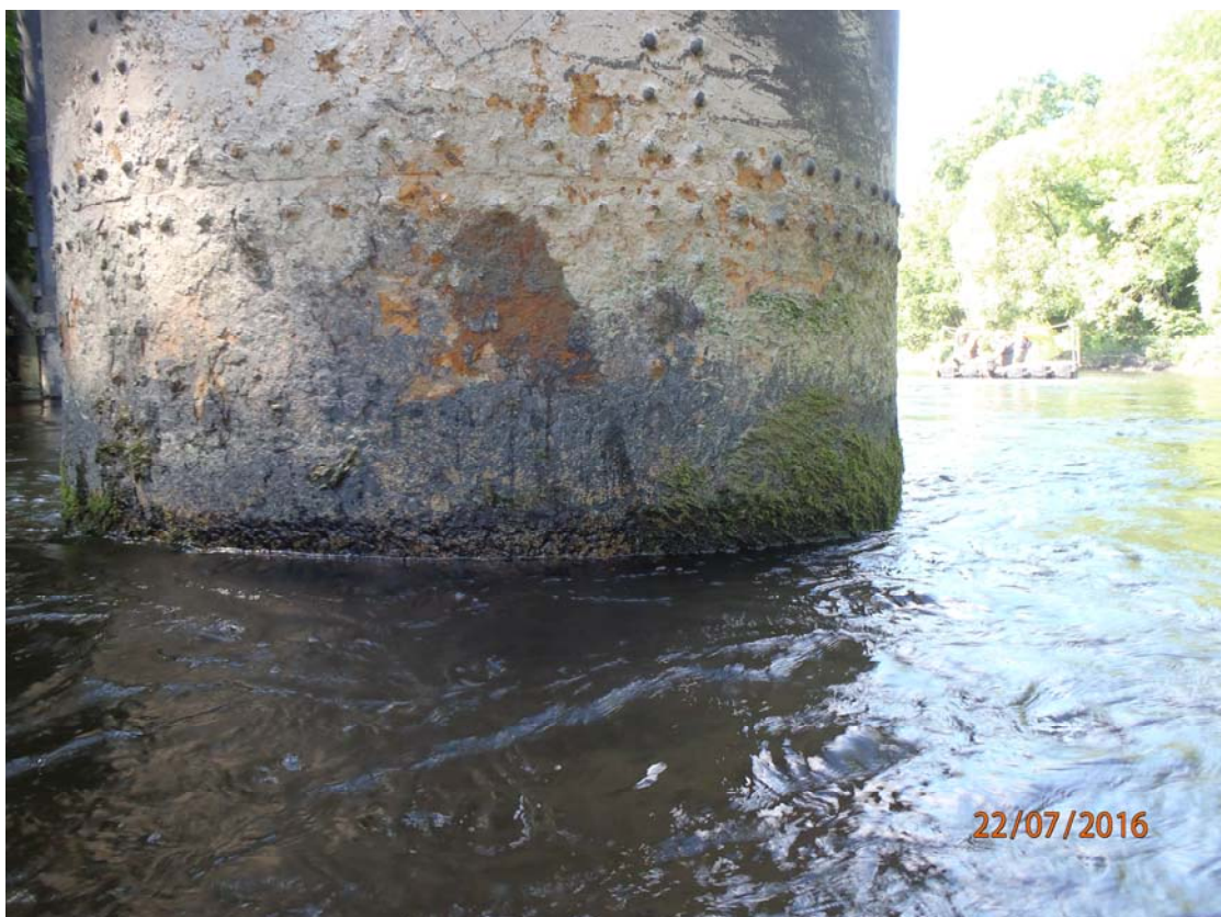
Photo 8 – View of Corrosion to Upstream Cylinder, Pier 4
