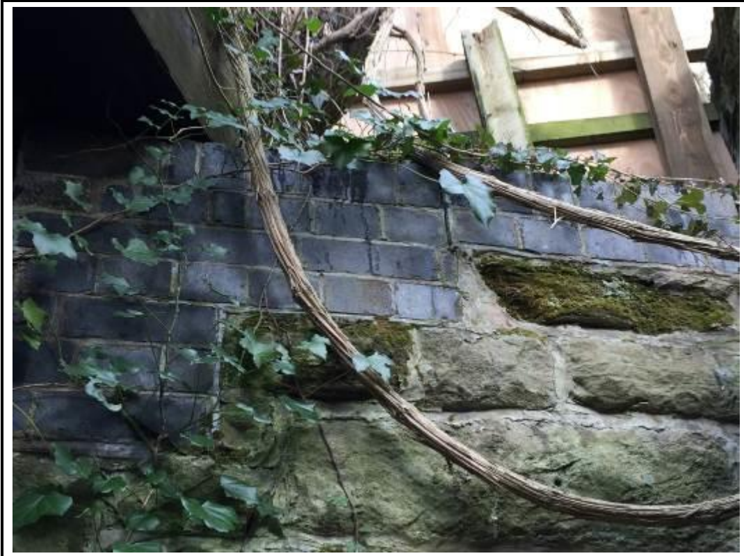
Photo 38. View of vertical fracture to high mileage abutment.
