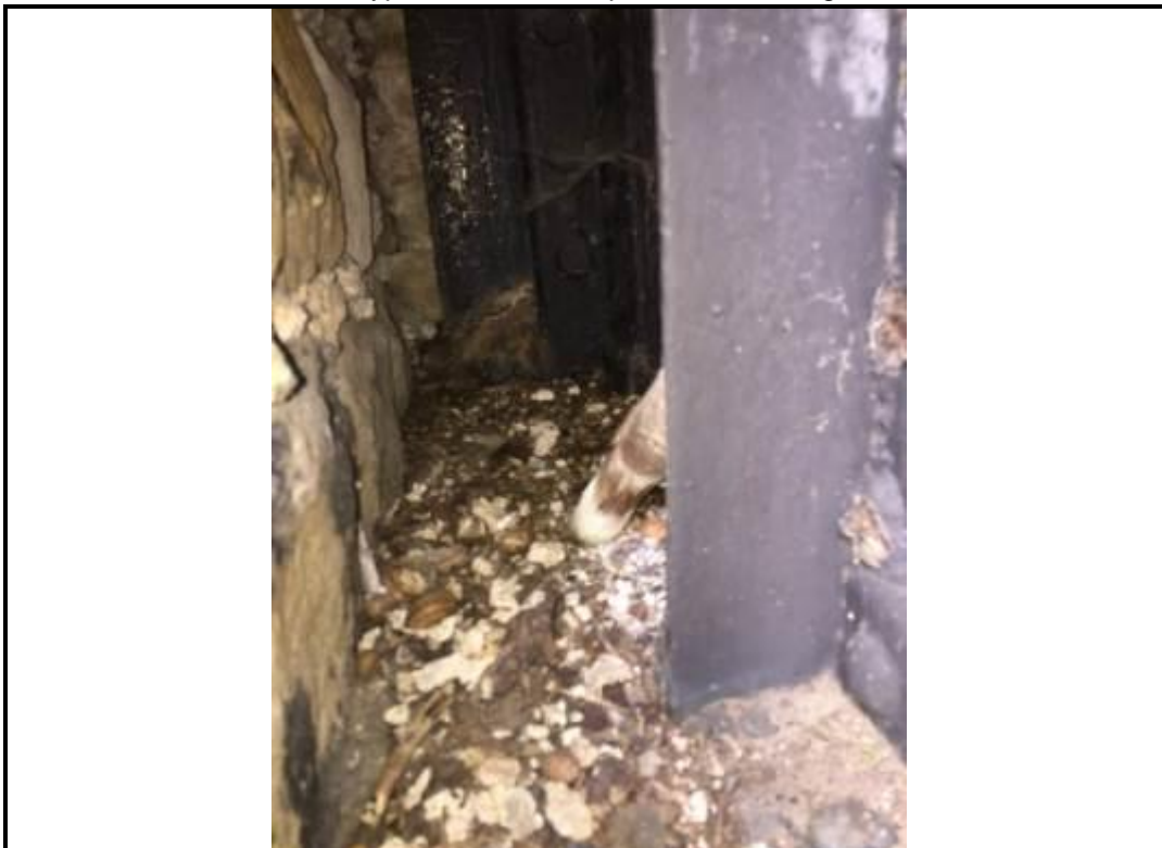
Photo 50. View of typical condition of bearing shelves.
