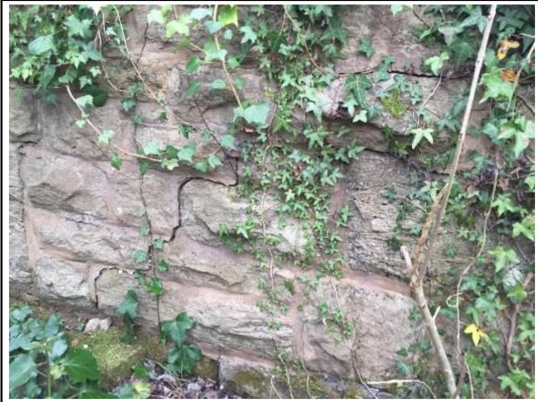
Photo 65. View of fracture to low mileage upside parapet.
