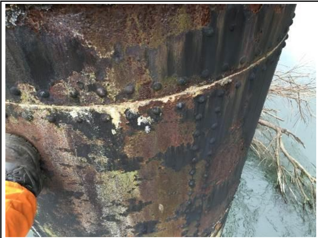
Photo 52. View of typical paint loss to piers 4 and 5.
