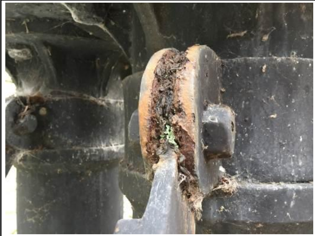
Photo 49. View of typical condition of pier cross bracing connections.
