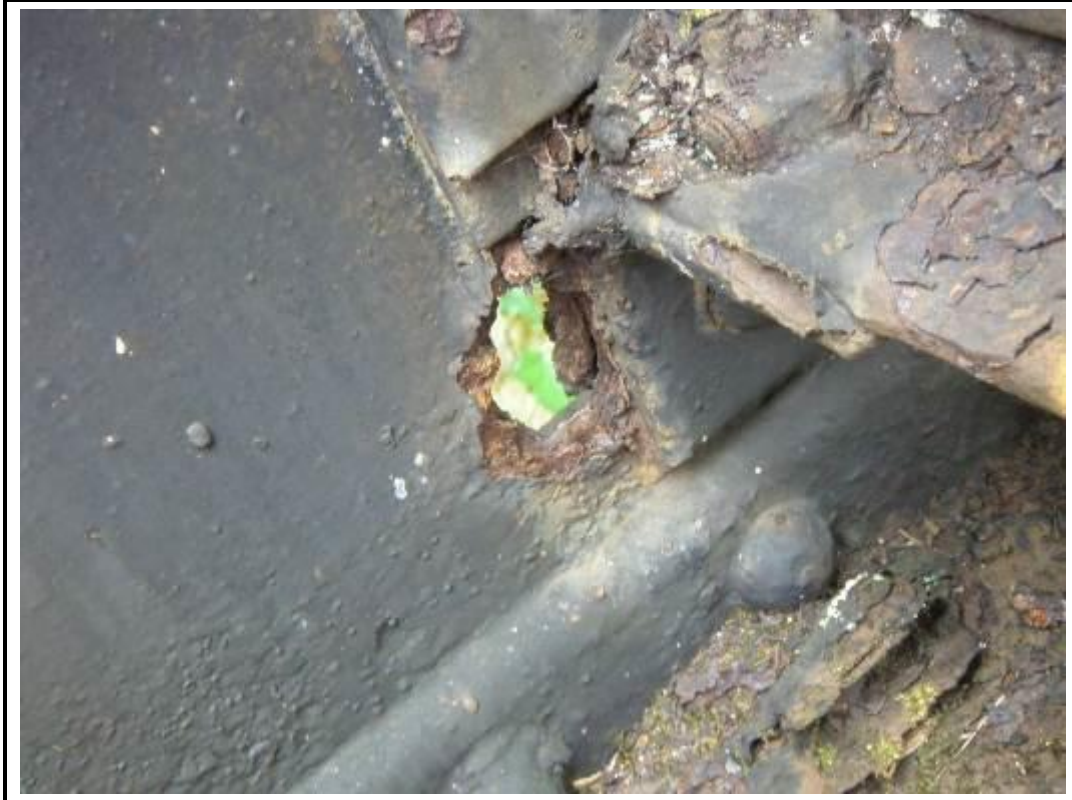
Photo 15. View of loss of section to web of transverse beam.
