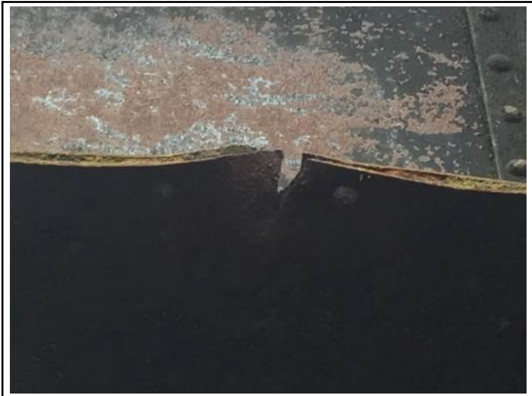
Photo 10. View of impact damage to downside beam, low mileage end.
