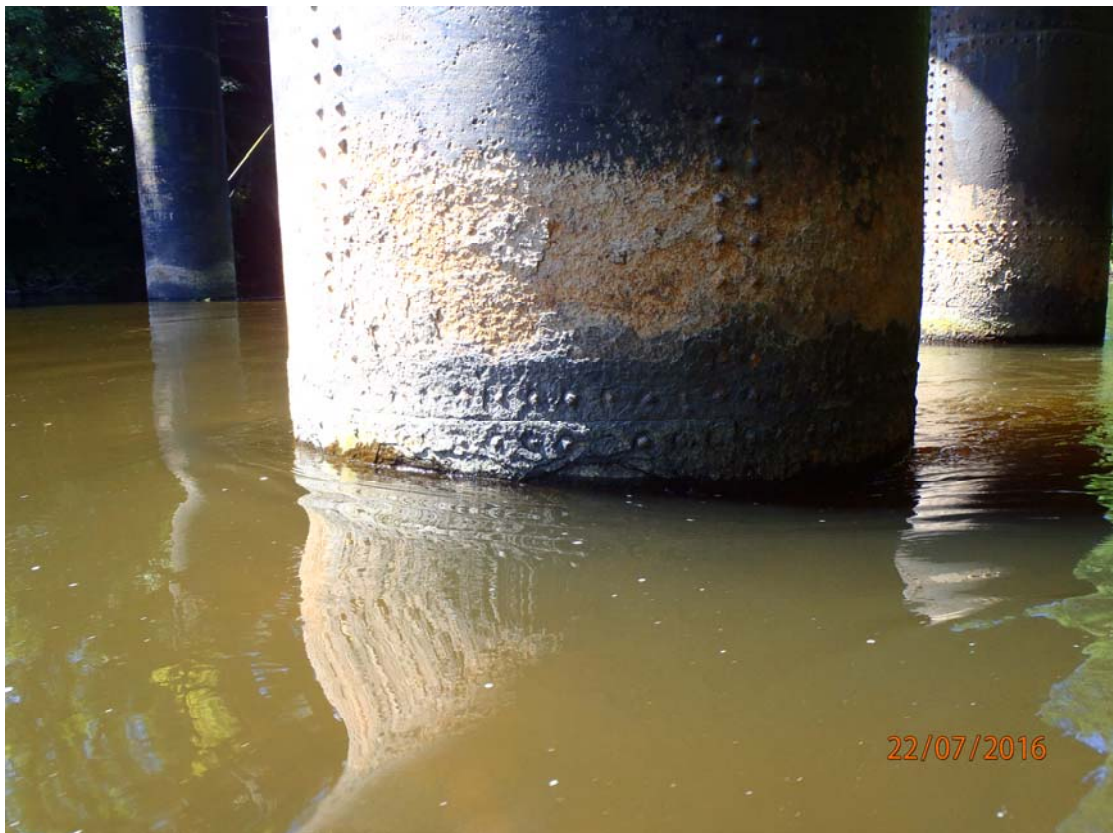
Photo 10 – View of surface corrosion / protective paint loss Upstream Cylinder, Pier 5
