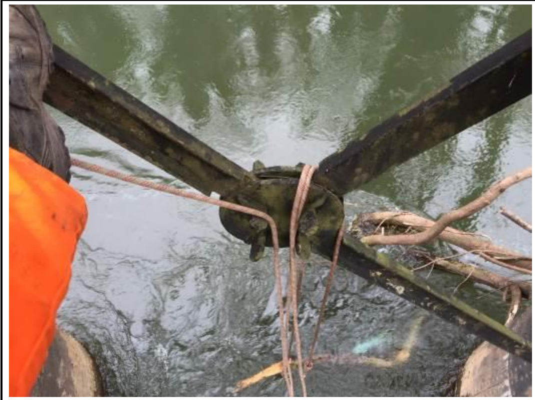
Photo 45. View of cross bracing between piers with missing lower tie.
