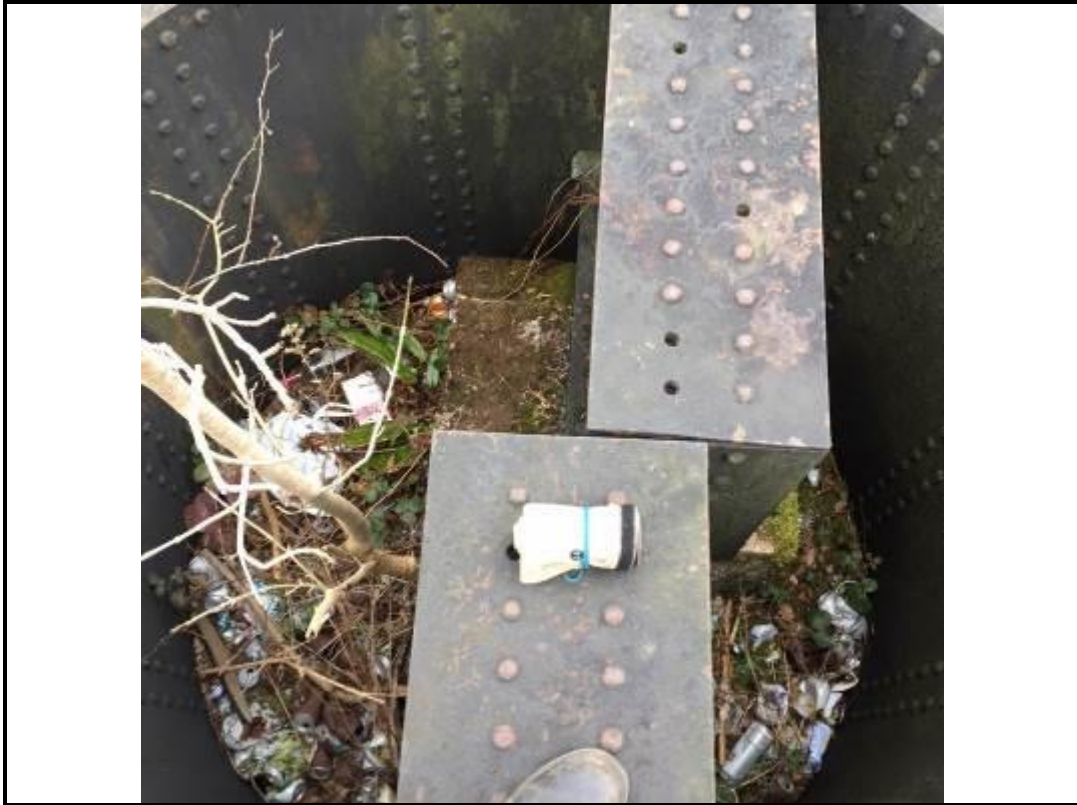
Photo 9. View of offset between two main girders, Pier 4 Upside Caisson.
