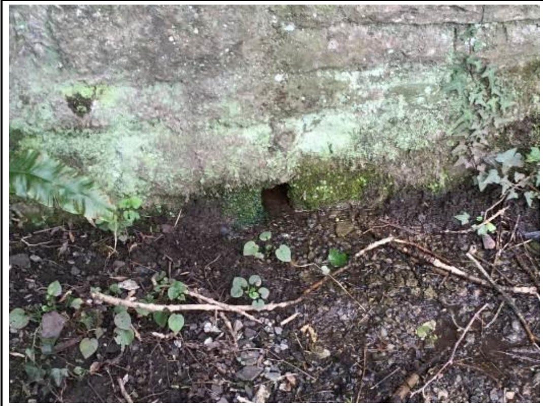
Photo 51. View of weep hole in high mileage abutment.
