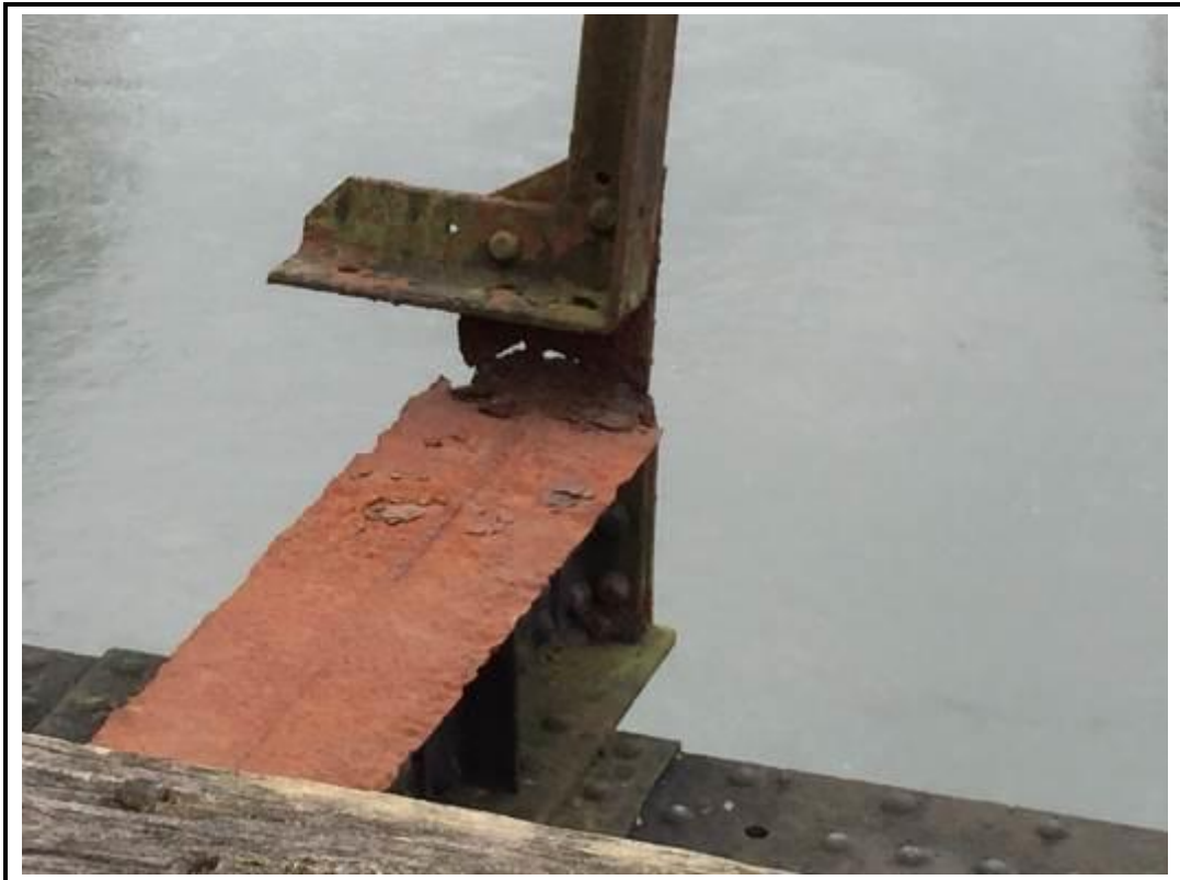
Photo 54. View of corrosion and LOS to base of handrail uprights.
