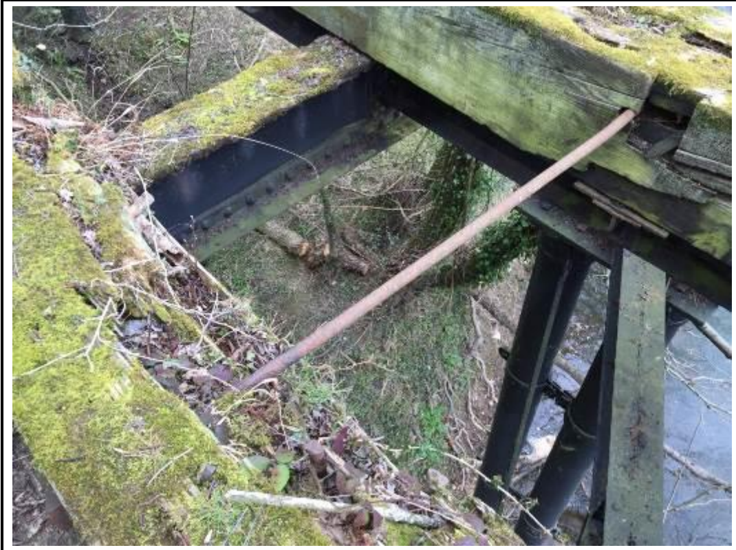
Photo 23. View of steel tie bar between timber baulks.
