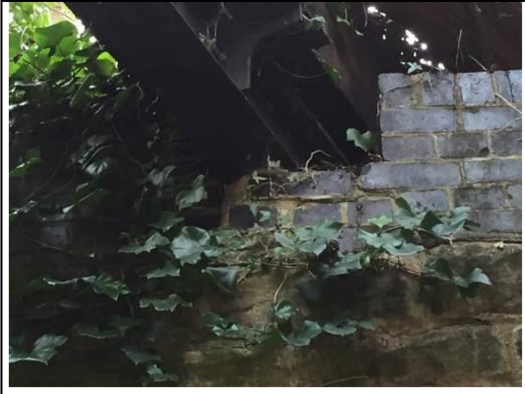
Photo 33. View of vertical fracture and displacement to low mileage abutment.
