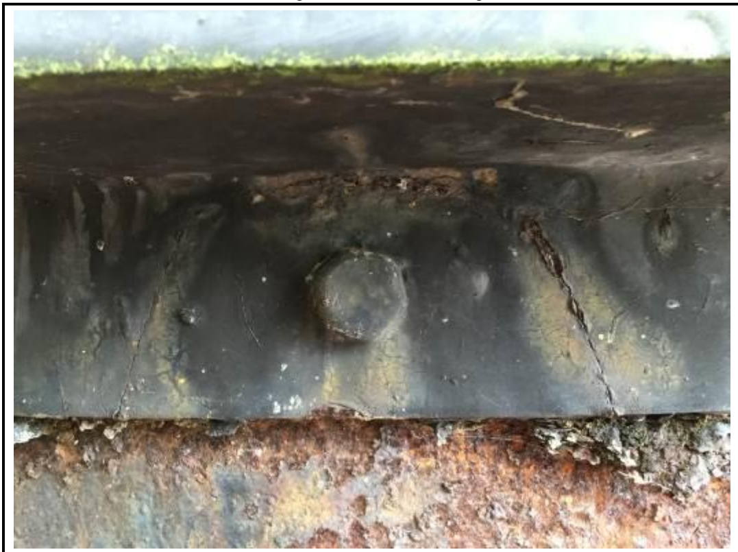
Photo 44. View of fracturing to pier 5 caisson decorative banding.
