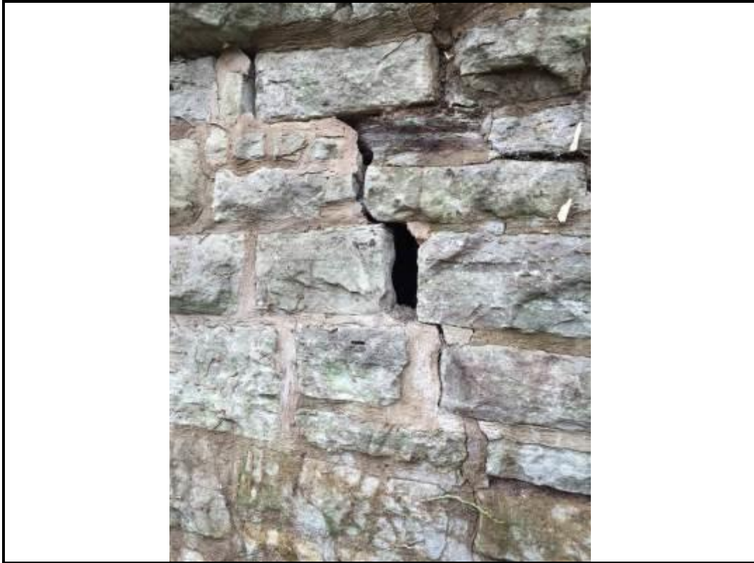
Photo 35. View of vertical step fracture to LM ABT downside return.
