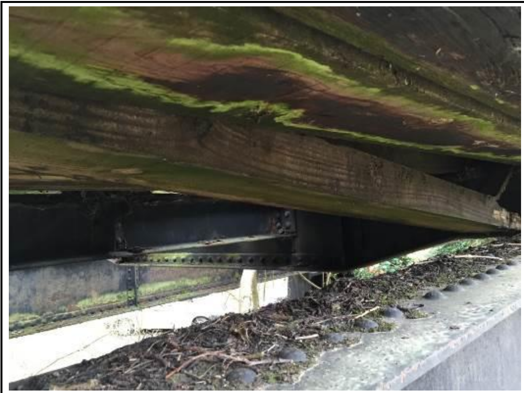
Photo 28. View of collapsed walkway timber.
