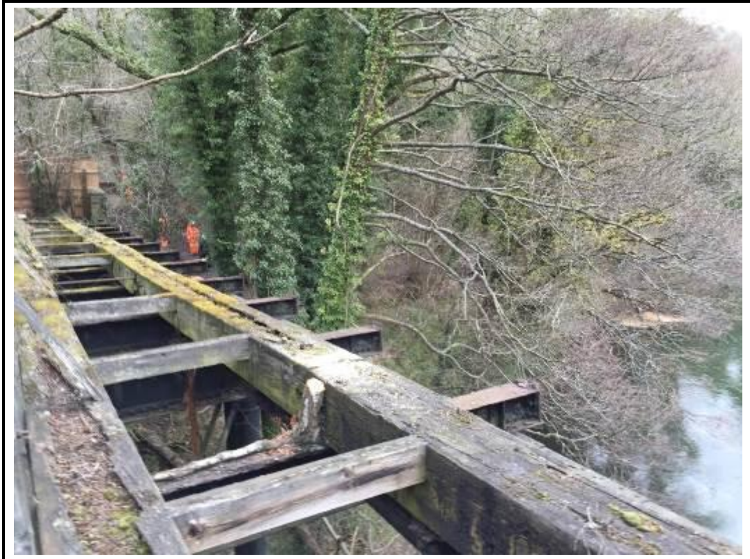
Photo 53. View of removed section of upside handrail.
