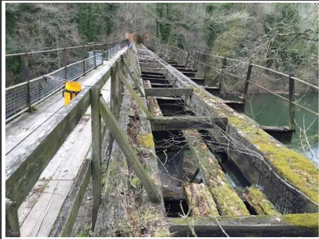
Photo 19. View of timber rail bearers.
