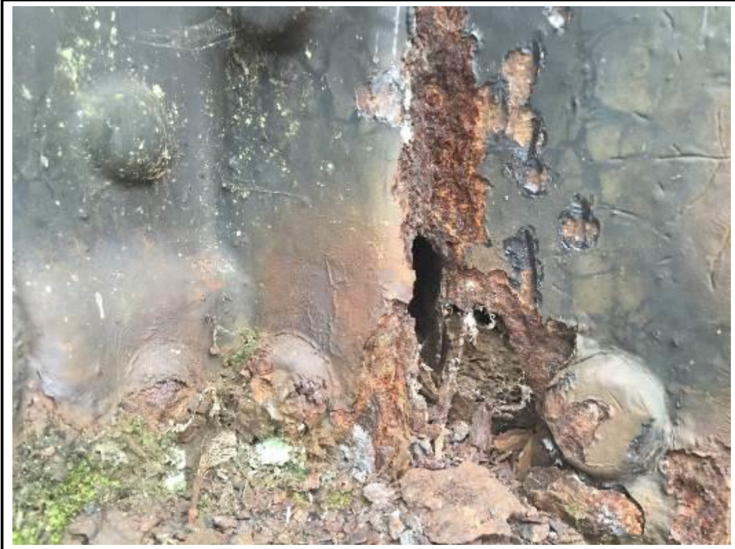
Photo 7. View of loss of section to gusset stiffener in MGE.
