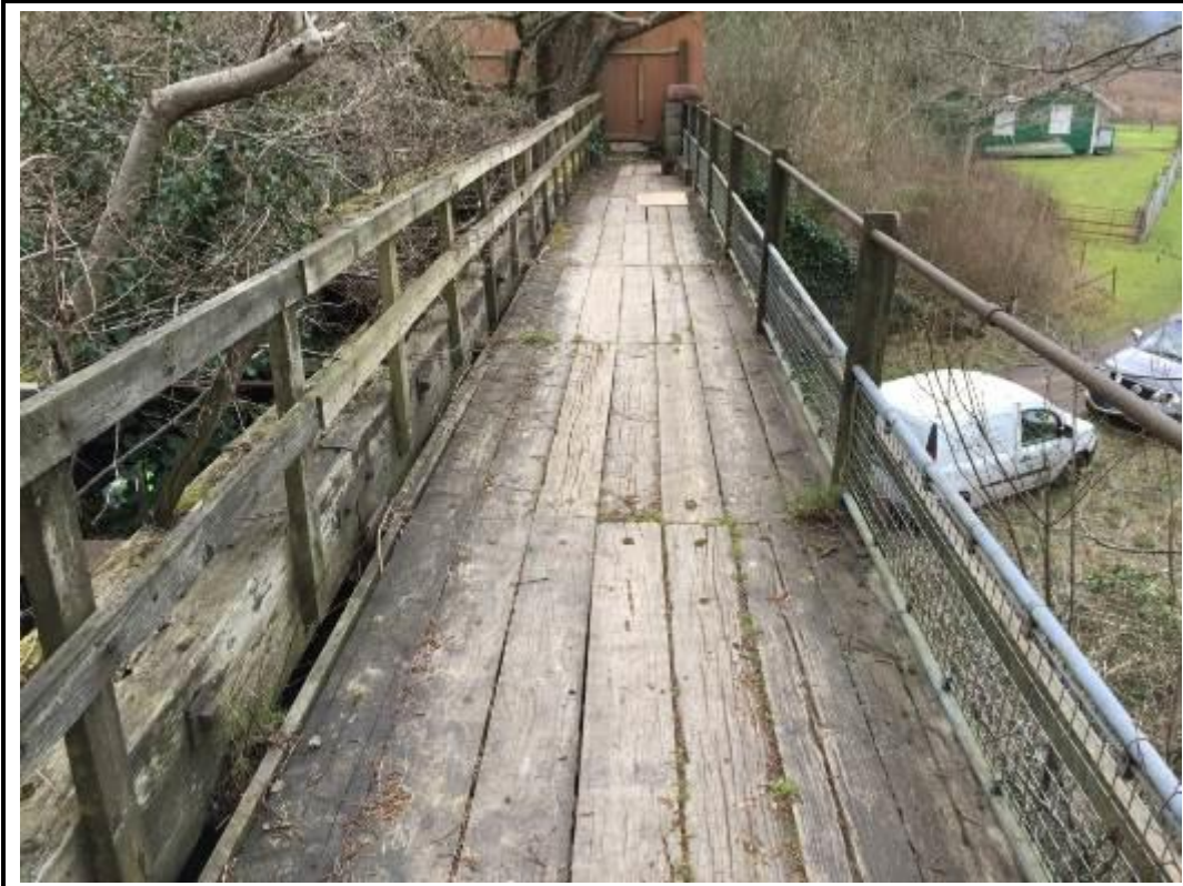
Photo 26. View of timber walkway planks.
