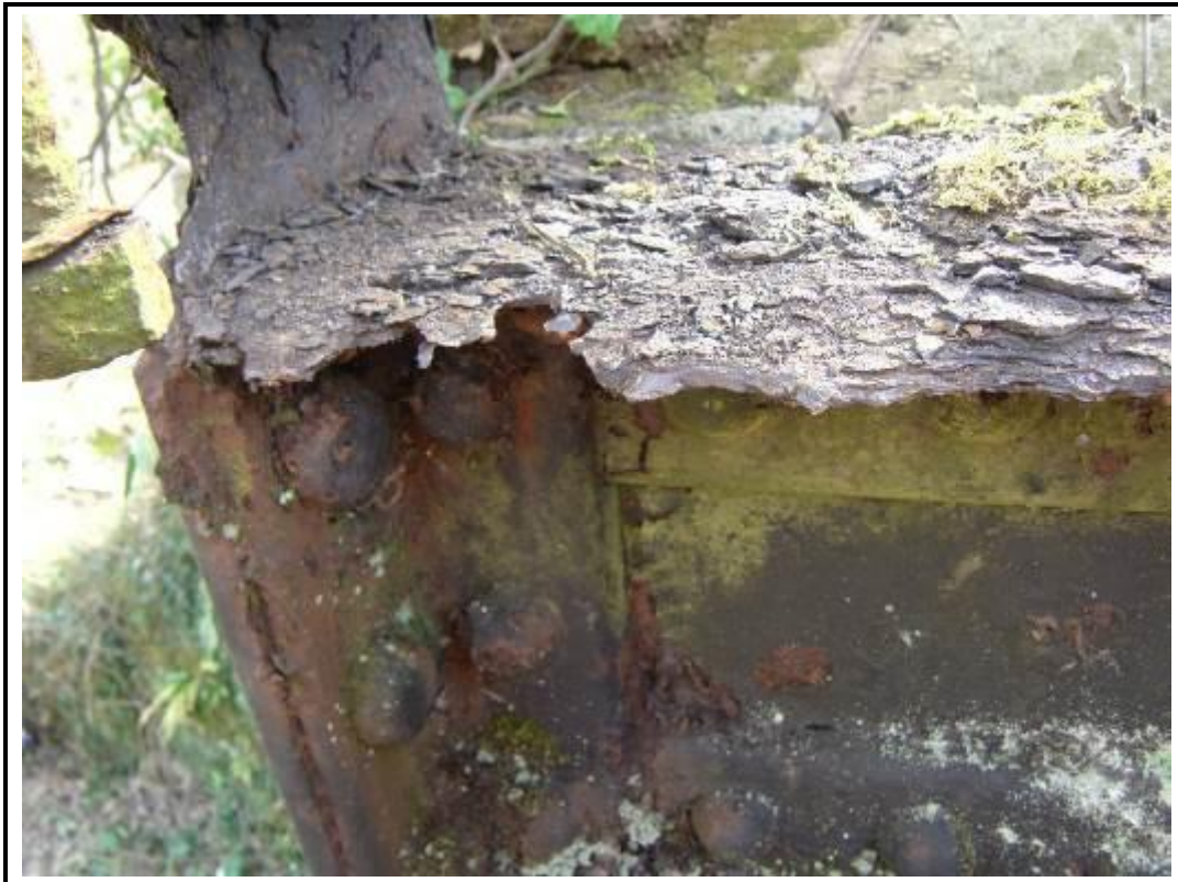
Photo 14. View of lamination, loss and knife edging to top flange, transverse beams.
