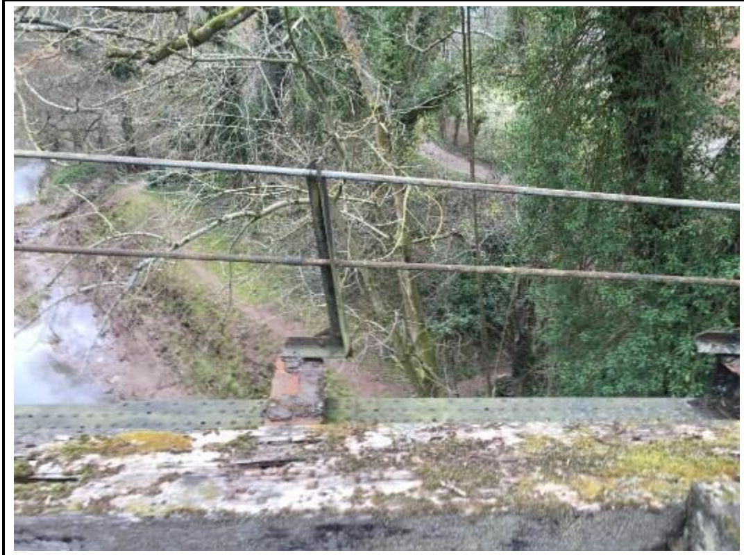
Photo 55. View of collapsed upright brackets on US handrail.
