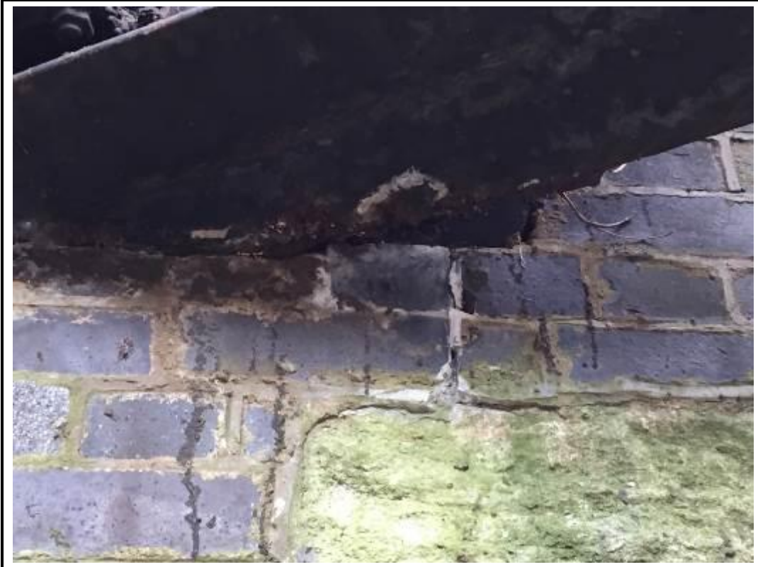
Photo 39. View of vertical fracture to high mileage abutment.
