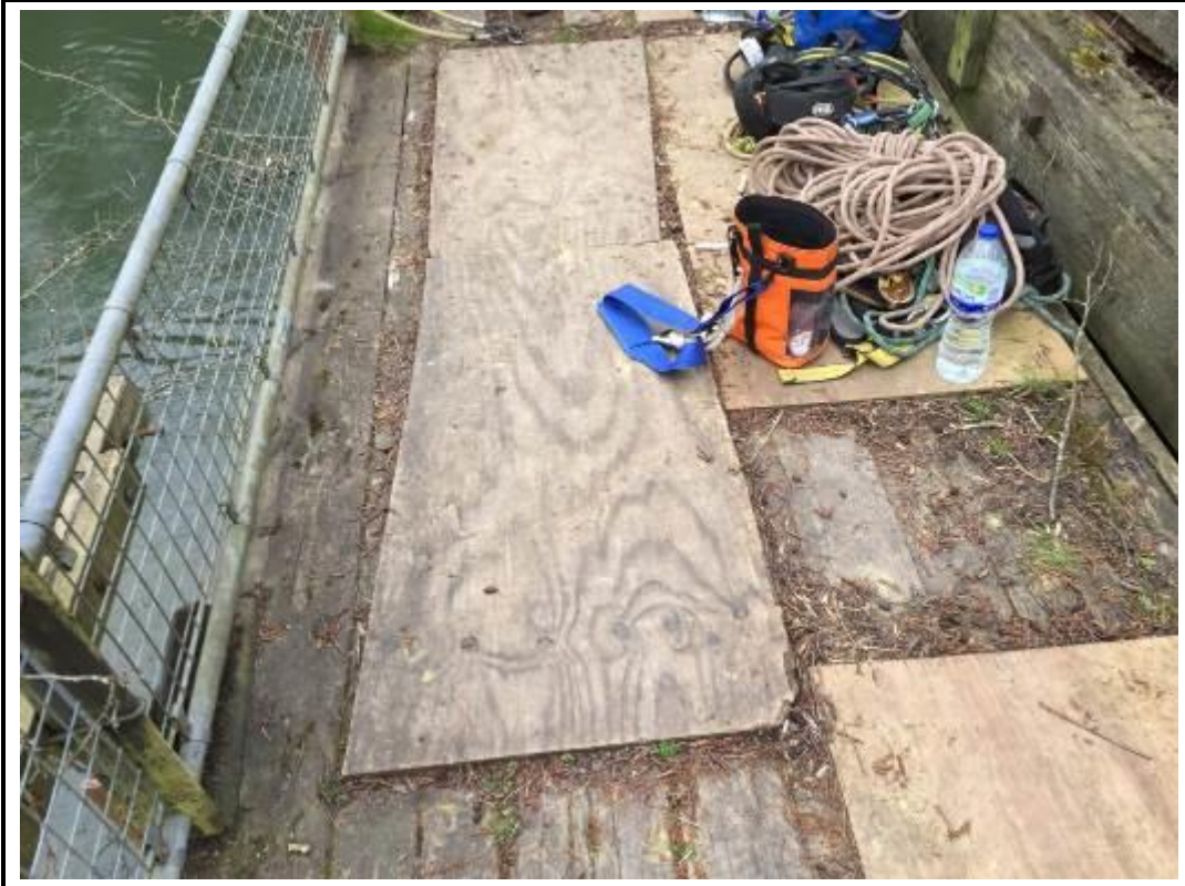
Photo 27. View of plywood repairs to walkway.
