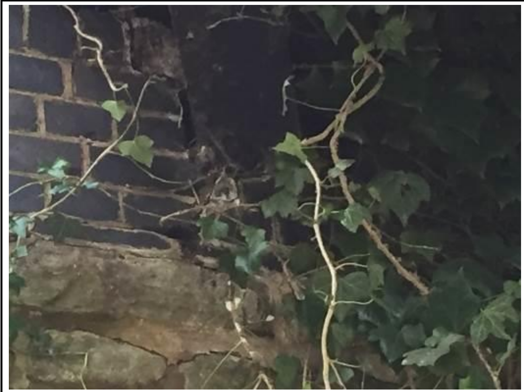
Photo 34. View of vertical fracture to low mileage abutment.
