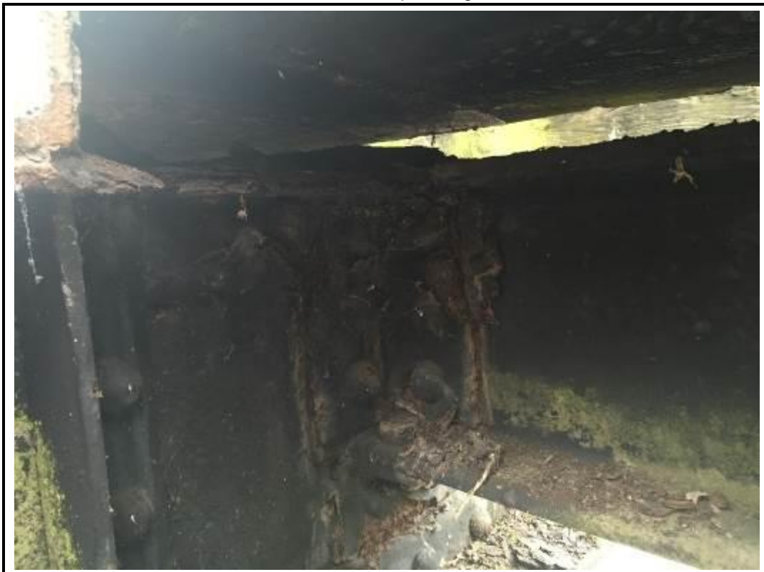
Photo 18. View of longitudinal beam corroded connection to transverse girder.
