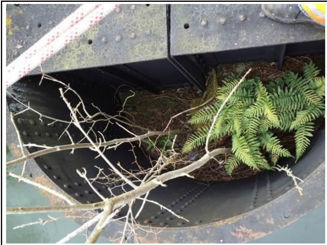
Photo 42. View of typical vegetation growth within caissons.
