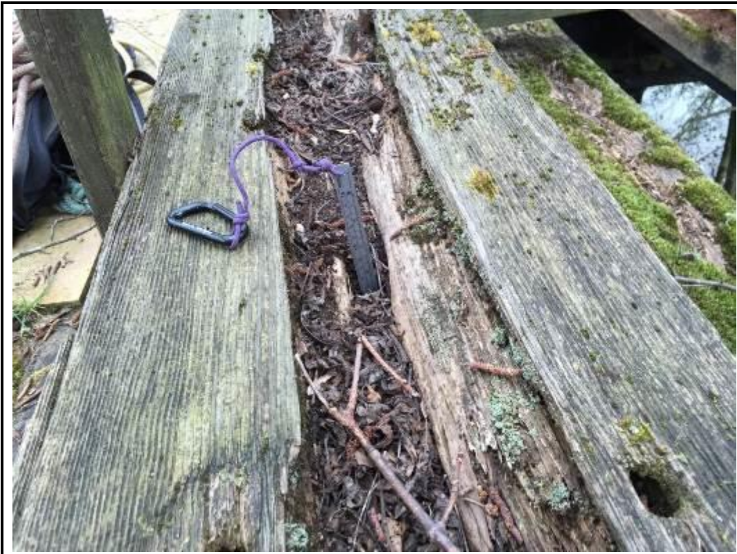
Photo 20. View of loss of section and rotting to timber baulk.
