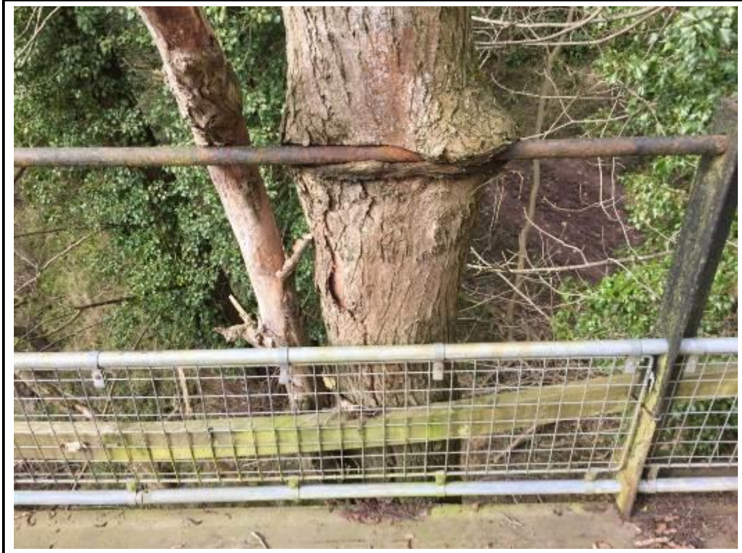
Photo 59. View of tree growth affecting downside handrail.
