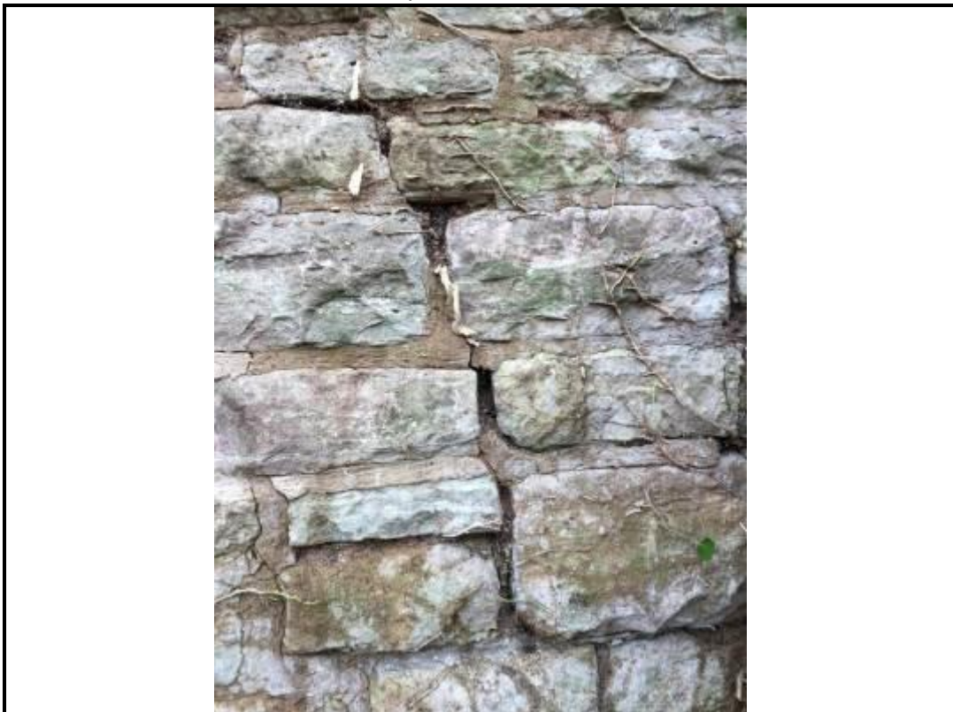
Photo 36. View of vertical fracture to LM ABT downside return
