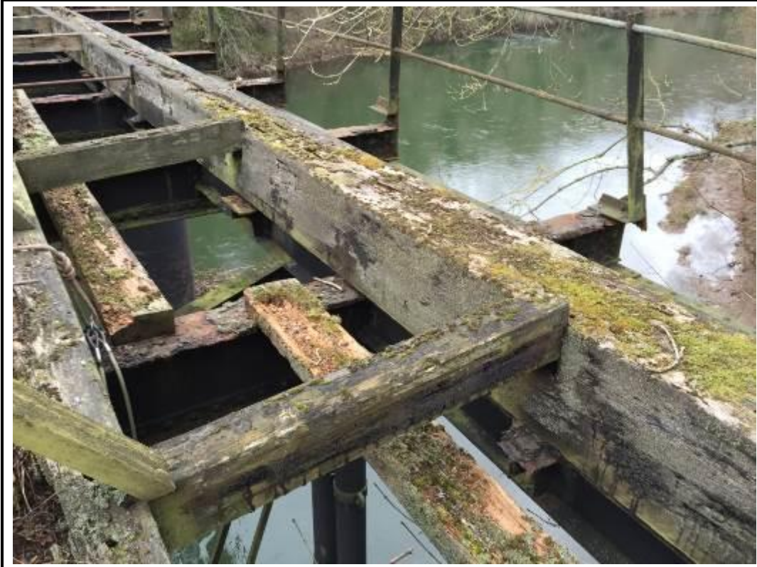
Photo 25. View of displaced cross timbers.
