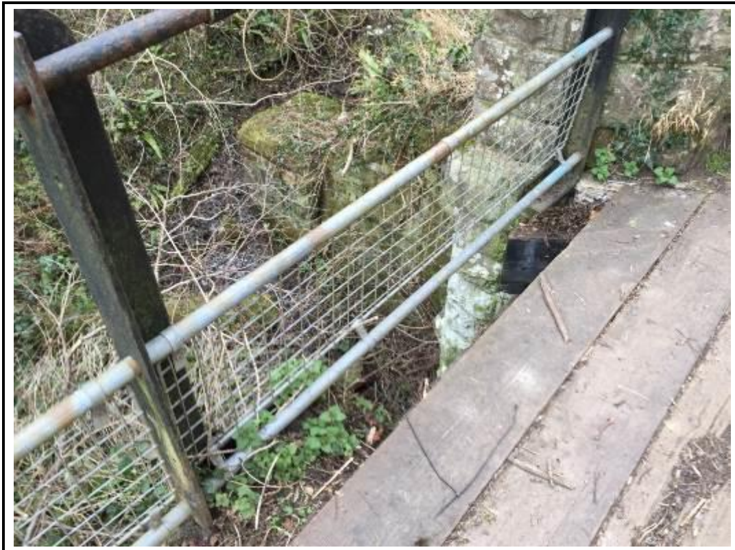
Photo 30. View of view of missing walkway timber at high mileage end.
