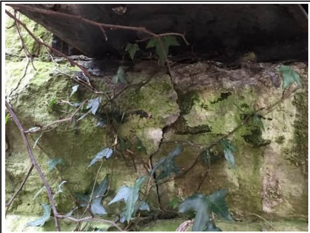
Photo 40. View of vertical fracture to high mileage abutment.
