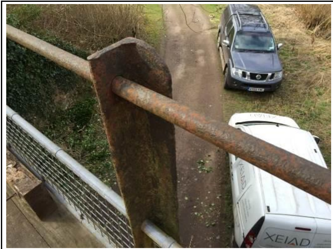
Photo 56. View of corrosion and pitting to downside handrail.
