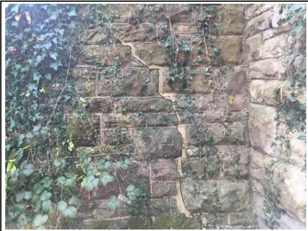
Photo 66. View of fracture to low mileage upside wing wall.
