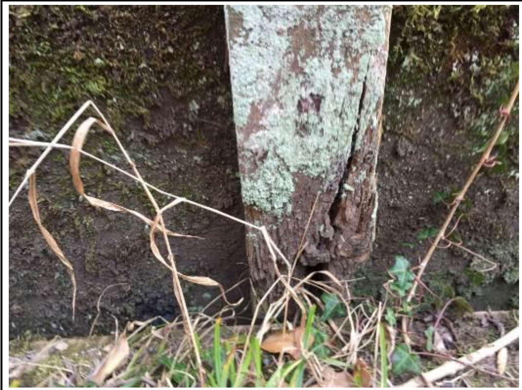
Photo 62. View of typical splitting to base of timber handrail.
