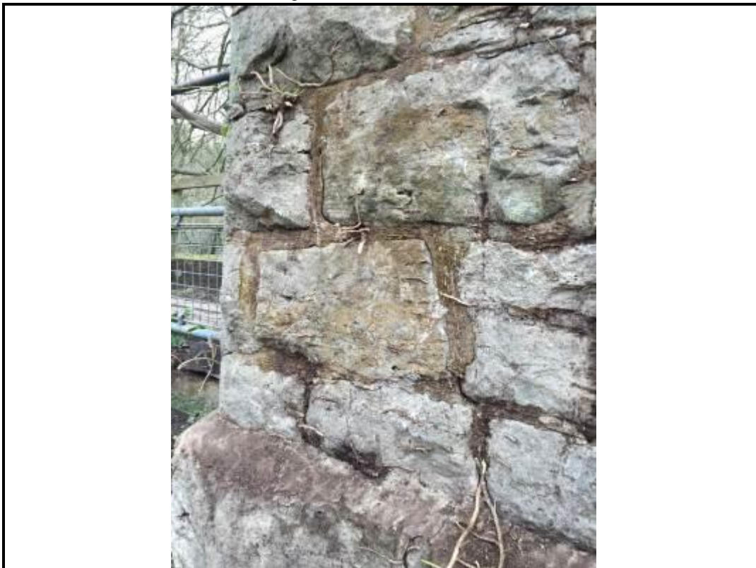
Photo 64. View of fracture to low mileage downside parapet.
