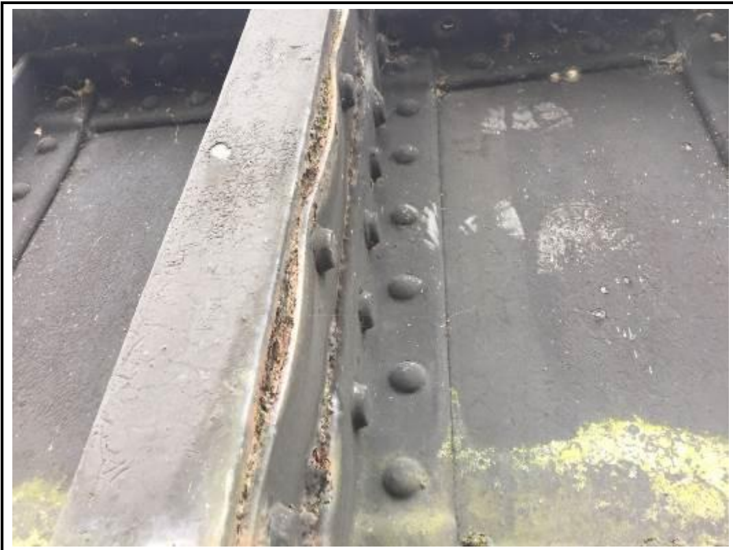
Photo 6. View of rust jacking to MGE upright stiffener plate
