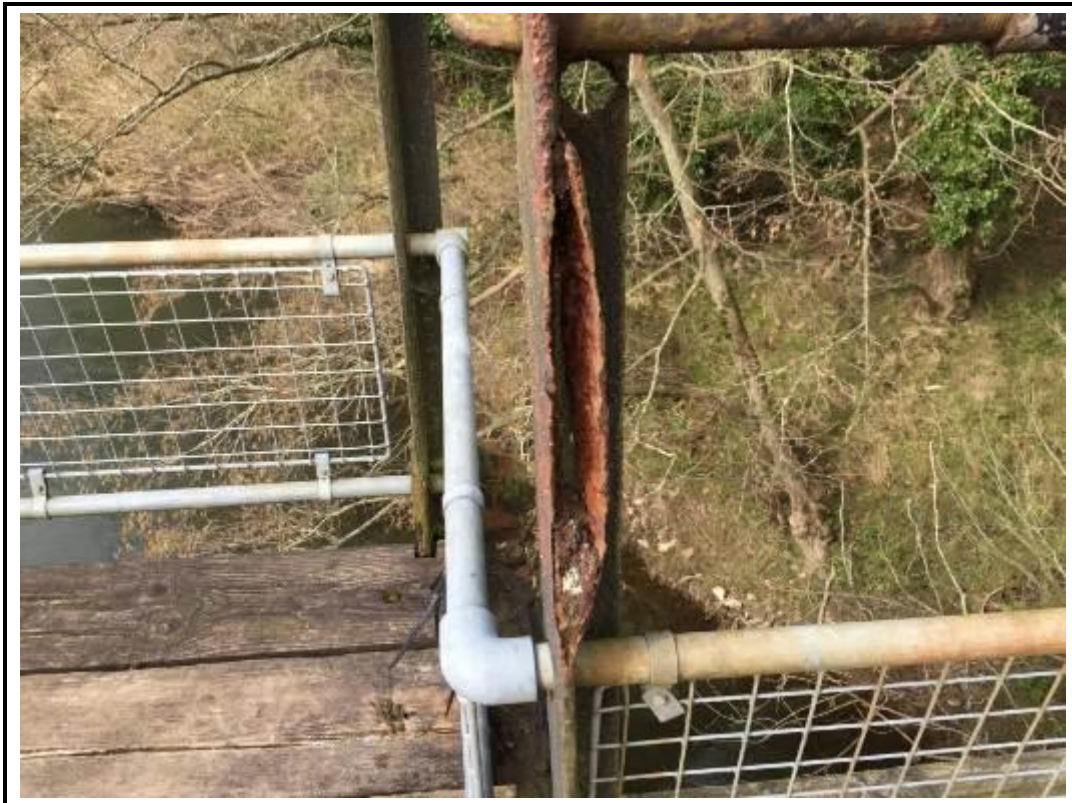
Photo 58. View of rust jacking to downside handrail upright.
