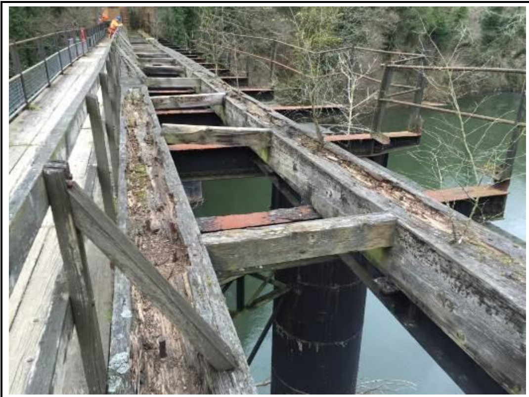
Photo 24. View of timber cross beams between timber baulks.
