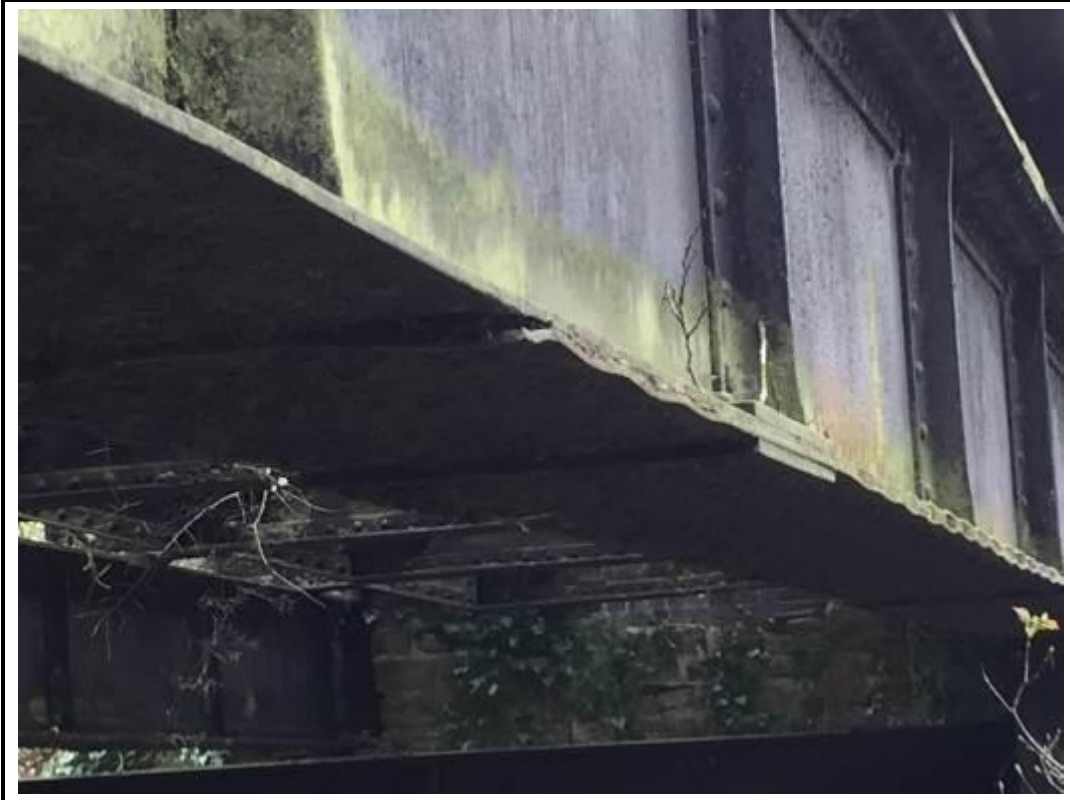
Photo 5. View of rust jacking to MGE bottom flange
