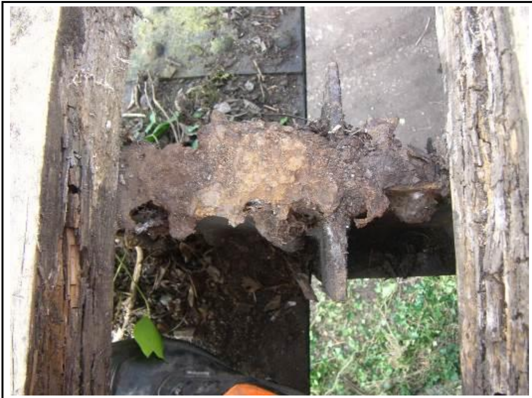
Photo 12. View of loss of section to transverse beams below walkway.
