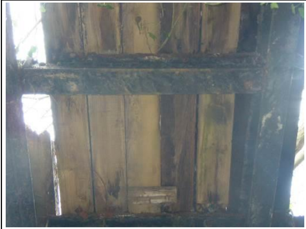
Photo 13. View of ineffectual timber clamps beneath walkway.
