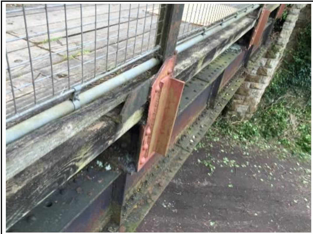
Photo 60. View of added bracing to downside handrail uprights.
