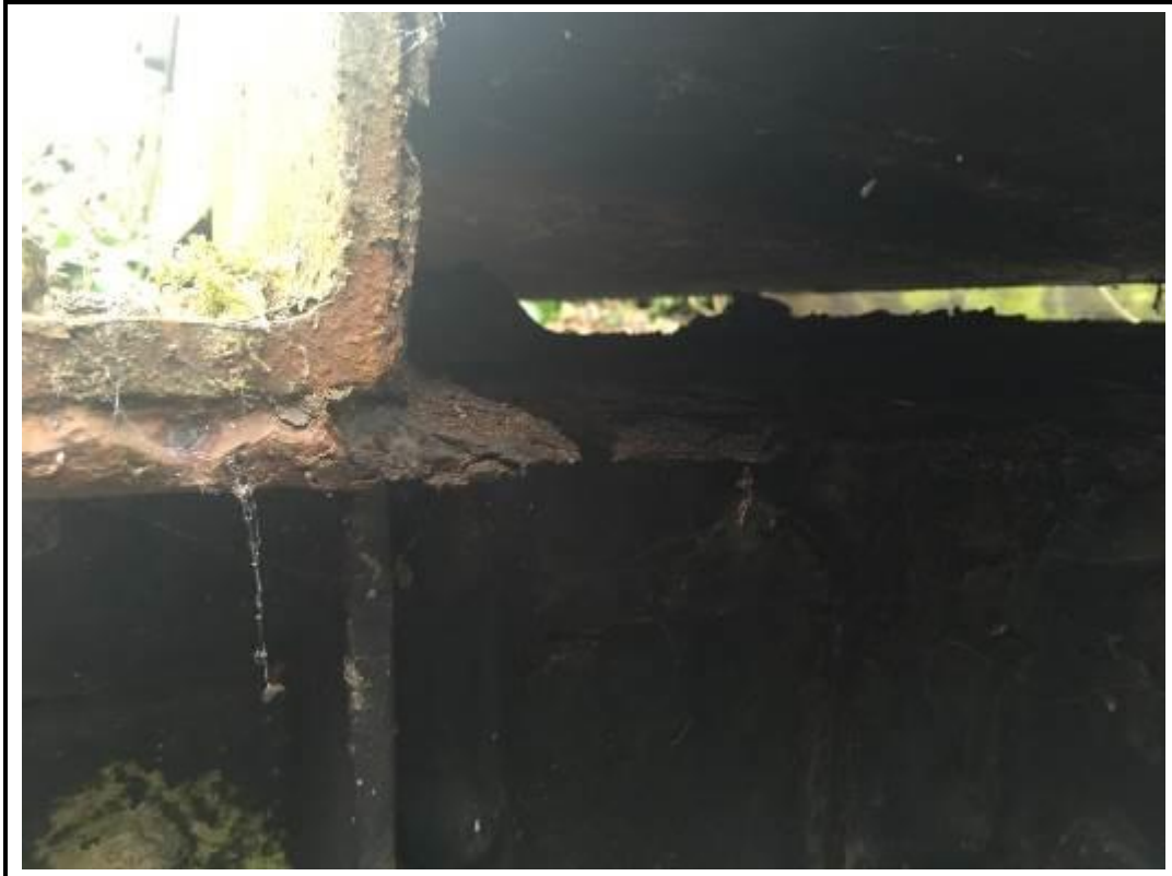
Photo 17. View of loss of section to top of longitudinal beams.
