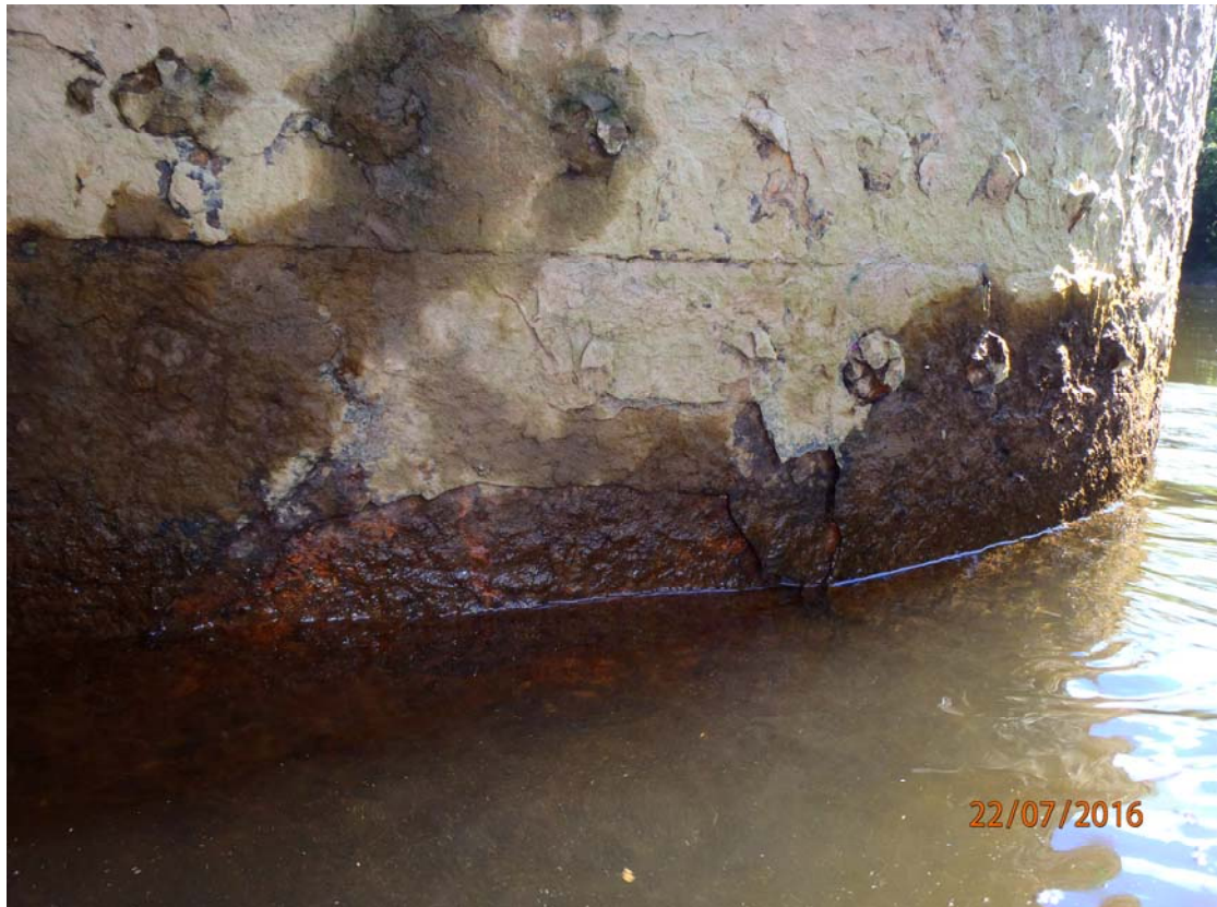
Photo 11 – View of surface corrosion Downstream Cylinder, Pier 5
