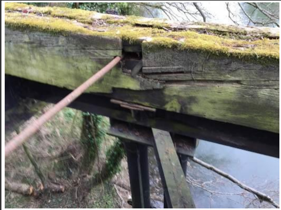
Photo 21. View of splitting to timber baulk.
