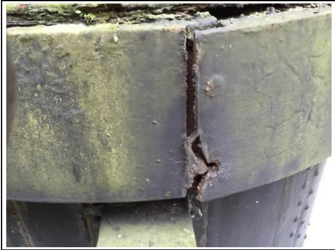
Photo 43. View of fracturing to decorative banding on caissons.
