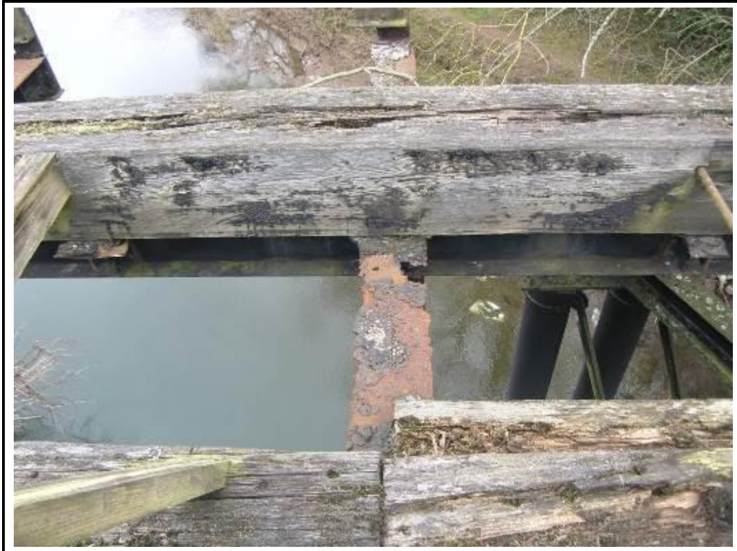
Photo 11. View of general loss of section to transverse beams top flange.
