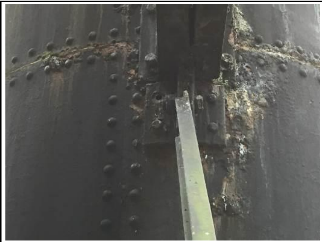
Photo 46. View of loose connector plate with missing bolt.
