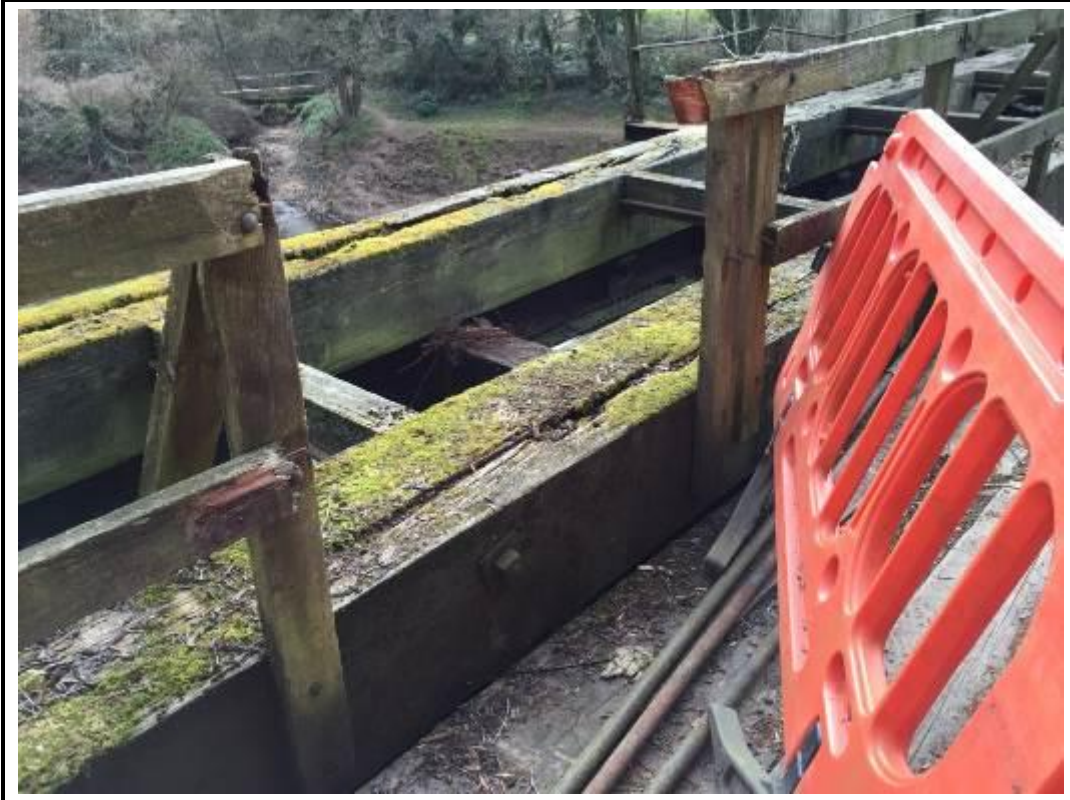
Photo 63. View of missing section to timber handrail.
