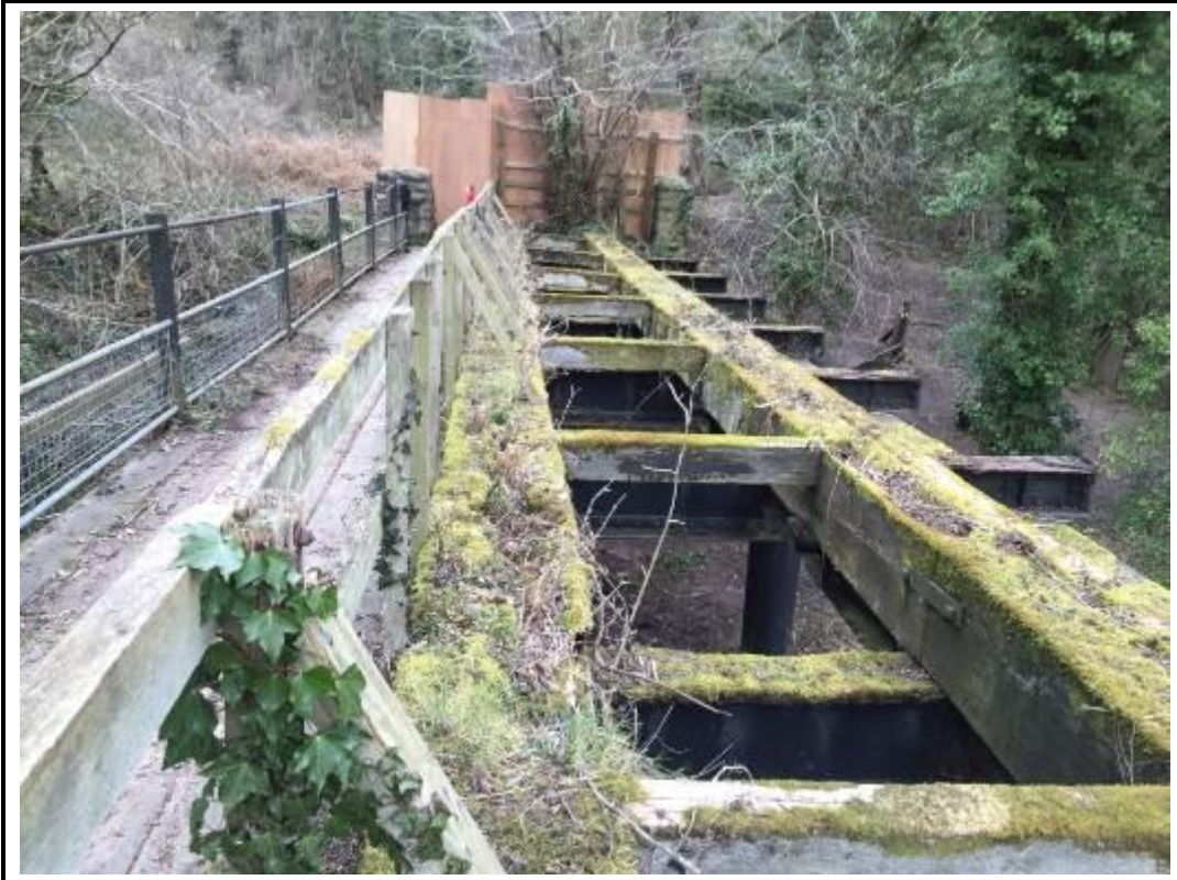
Photo 22. View of vegetation growth on timber baulks.
