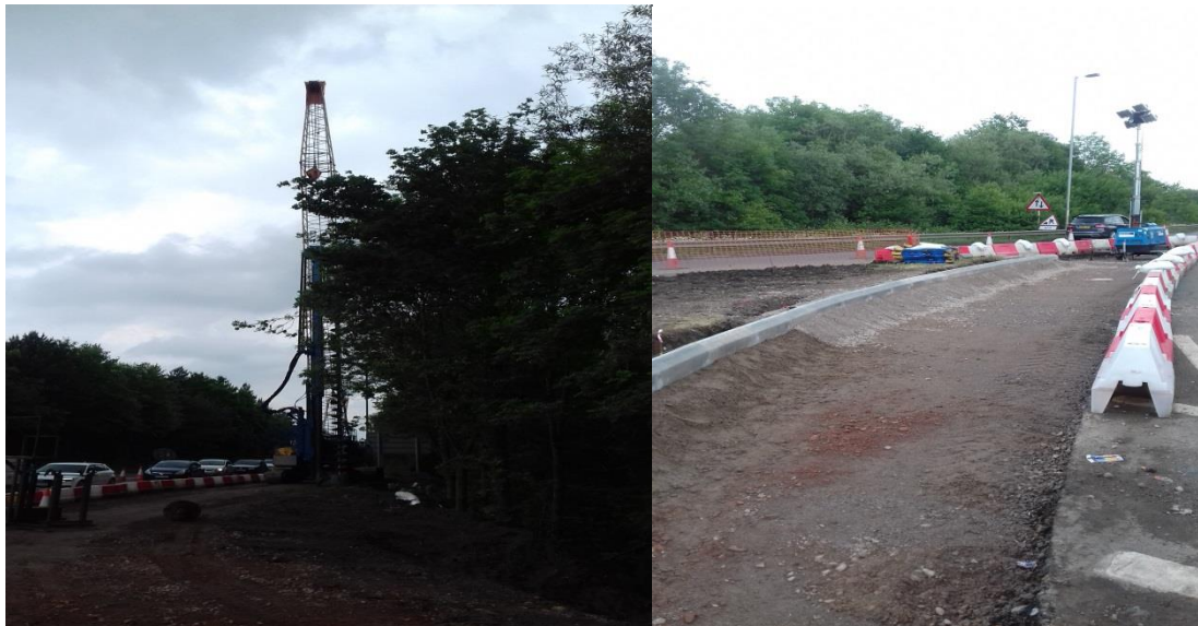
Plant, for the installation of the sheet piles on the A417 Southbound. Kerbing on A40 Westbound
