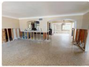
Homeowners Hurricane Documentation
