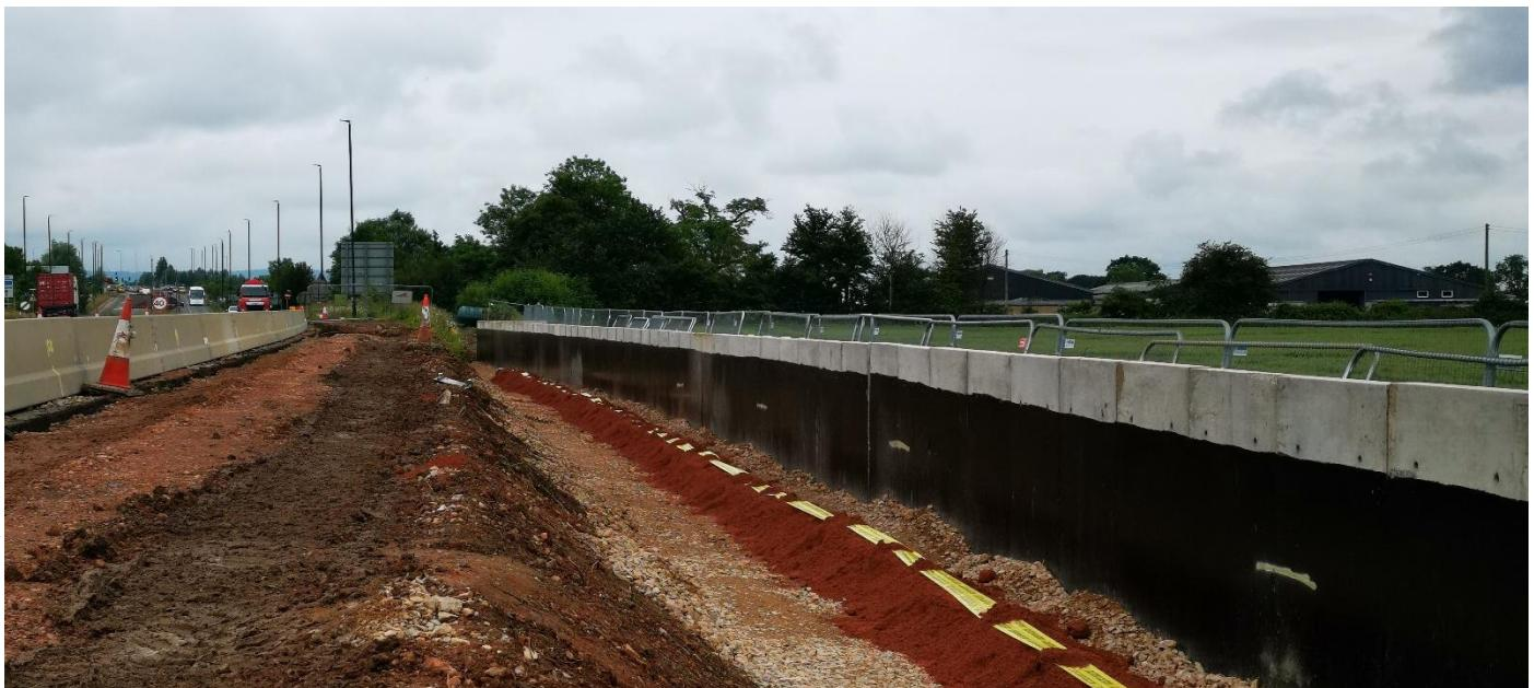
We've completed the temporary surface on the inside lane of the roundabout and installed drains near the site of the old Cross Keys Pub. We've also set up a temporary safety barrier along the A38 approach to Cross Keys from Gloucester to keep crews safe.
