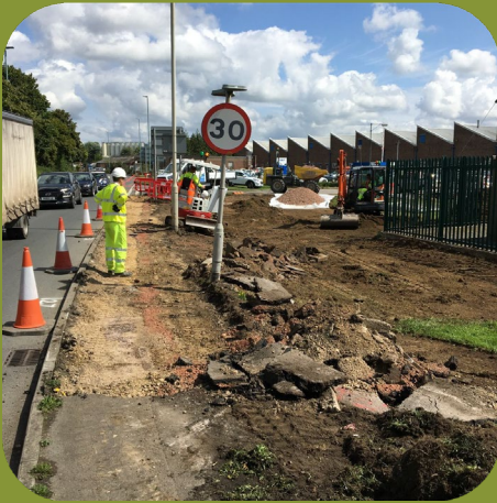
Stripping of Top Soil at Old Ends Lane
