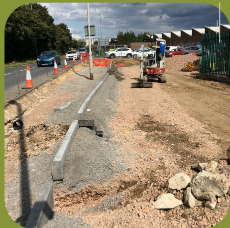
Installation of new kerb line at Old Ends Lane
