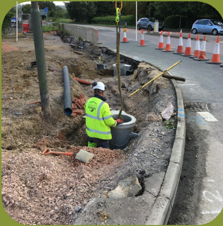
Installation of gully pots at Old Ends Lane
