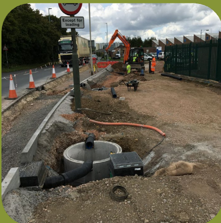
Drainage and manhole construction at Old Ends Lane
