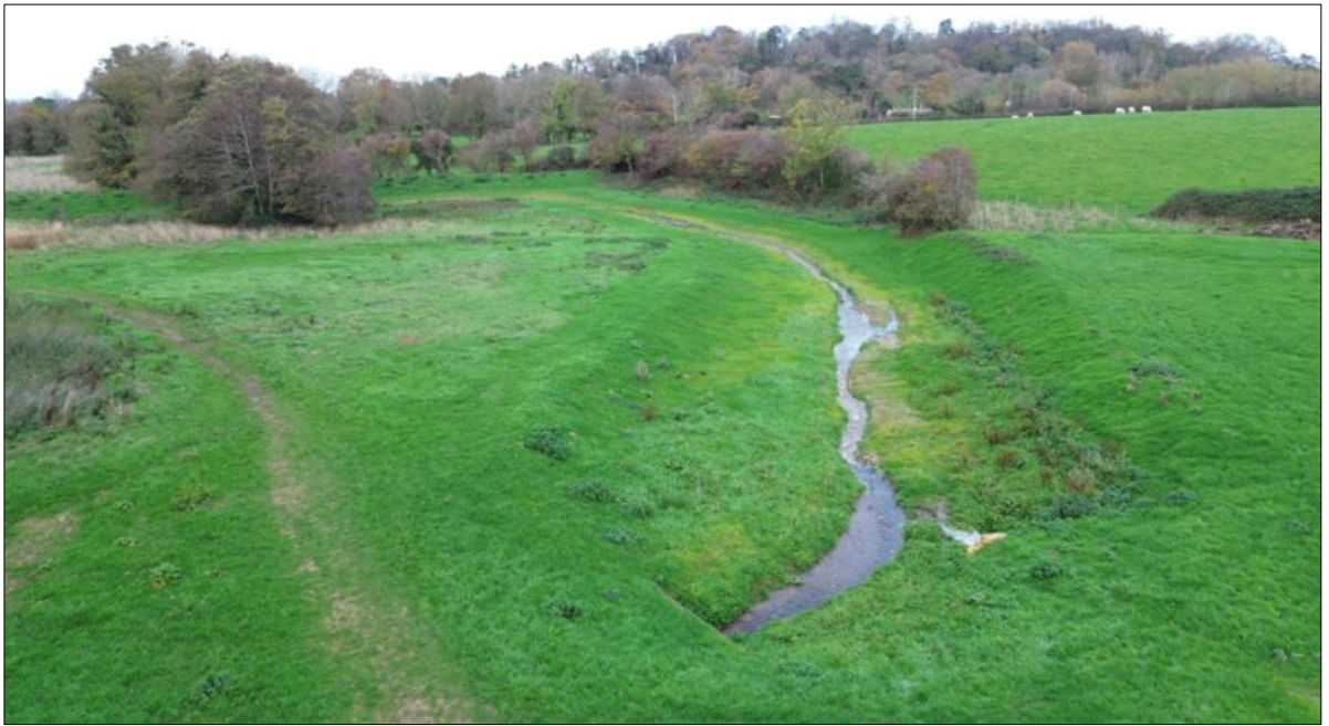
FAS viewed upstream to downstream
