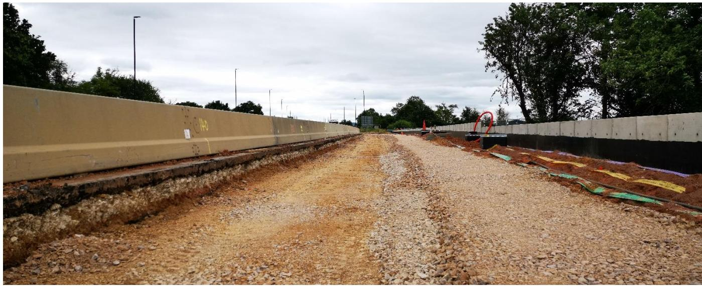
Works have started in the verge between the A38 approach from Whitminster/Stroud, and the A38 towards Gloucester from Cross Keys Roundabout. This has included removing street lighting, stripping the top layer of soil and starting construction on the carriageway. Barriers are in place for the safety of the crews.
