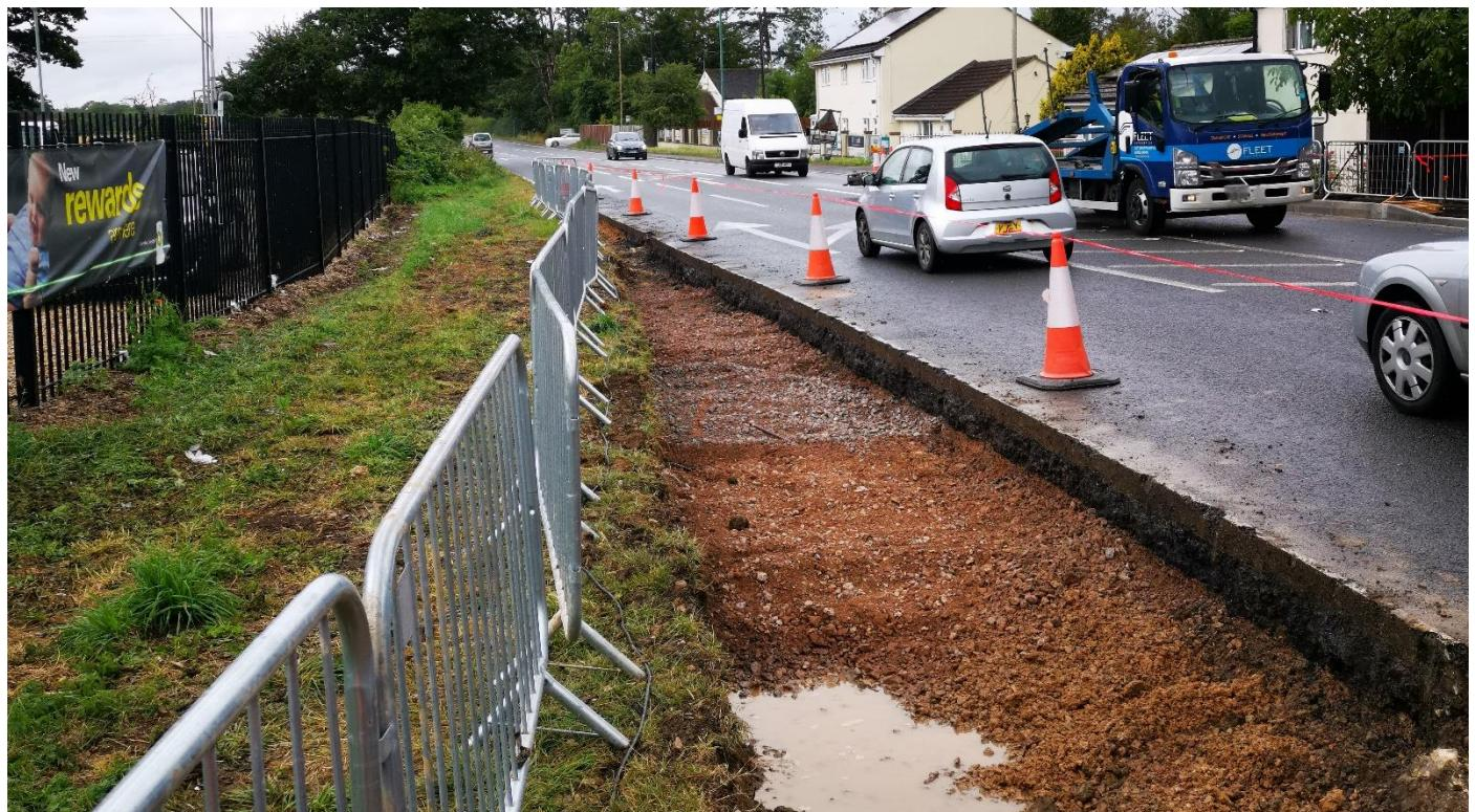
Works have continued in the verge between the A38 approach to Cross Keys Roundabout from Whitminster/Stroud and the A38 towards Gloucester from Cross Keys Roundabout, with the kerb alongside the new widened carriageway completed.
