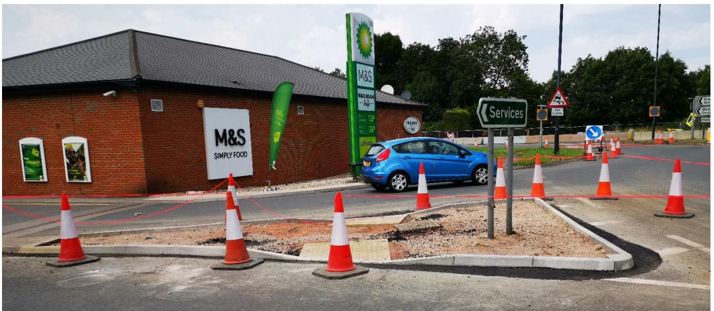
The drainage and kerbs will soon be complete where we are widening the carriageway as you head toward Whitminster/Stroud from Cross Keys Roundabout.
