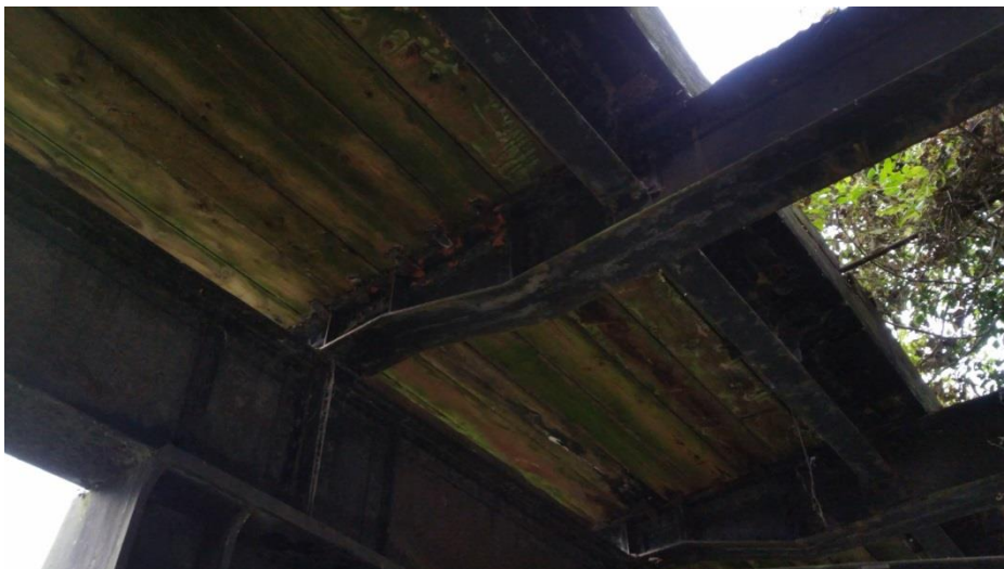
Picture 7 Transversal and secondary girders
