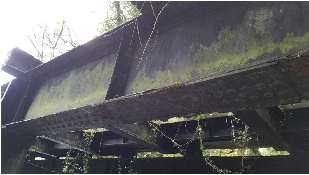
Picture 5 Detail of rust jacking on longitudinal girder
