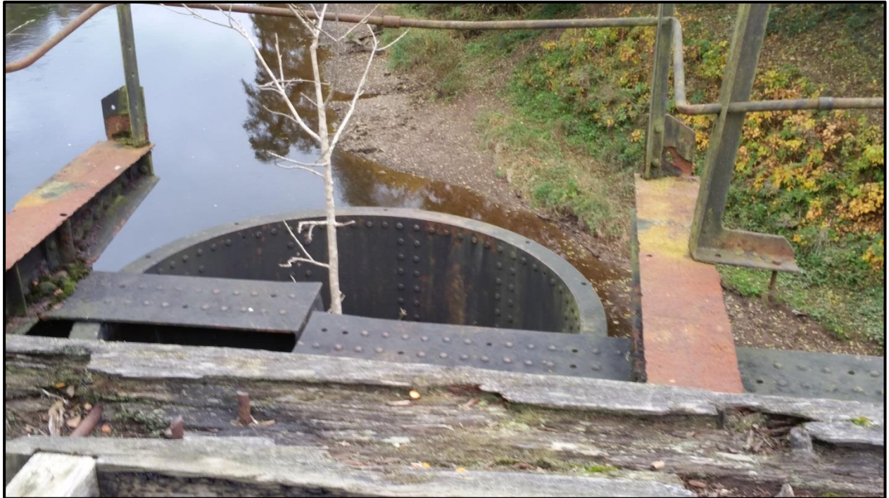
Picture 24. Main girders and caisson
