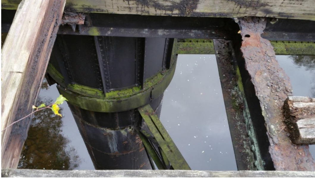
Picture 6 Detail of corrosion on top flange of transversal girder
