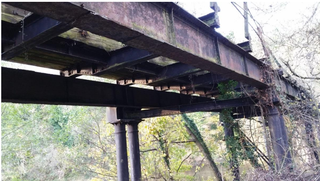
Picture 8 Cast Iron columns
