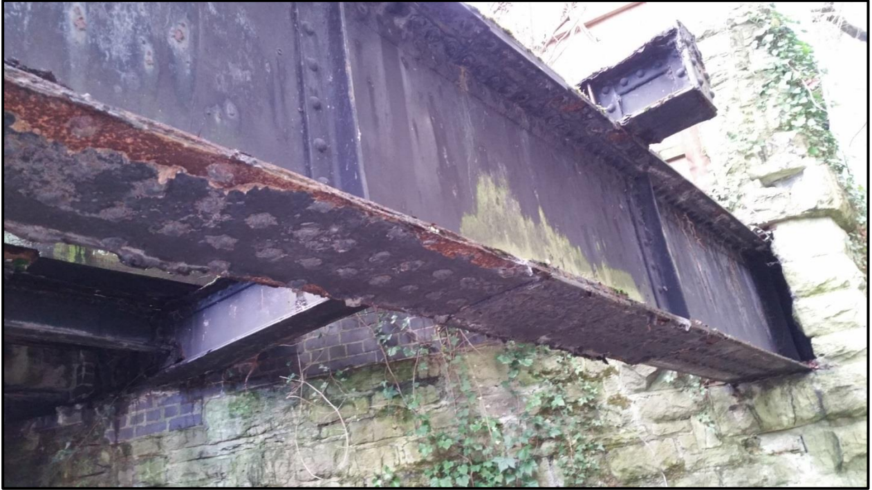
Picture 18. Main girder bottom flange
