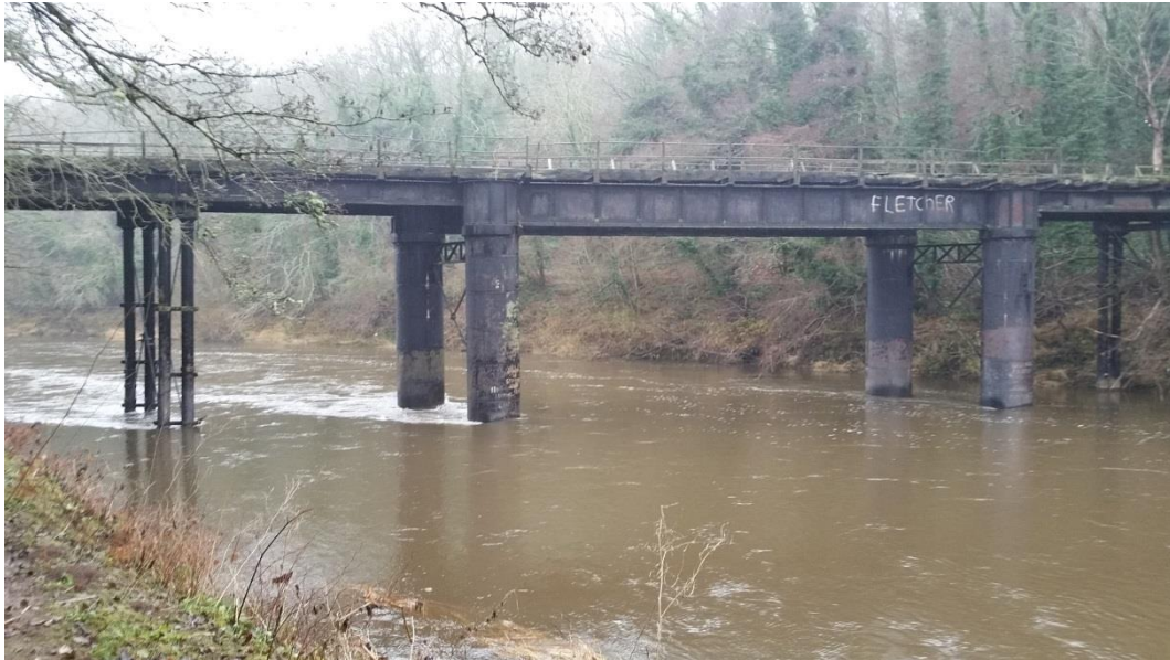
Picture 9 Caissons at central span
