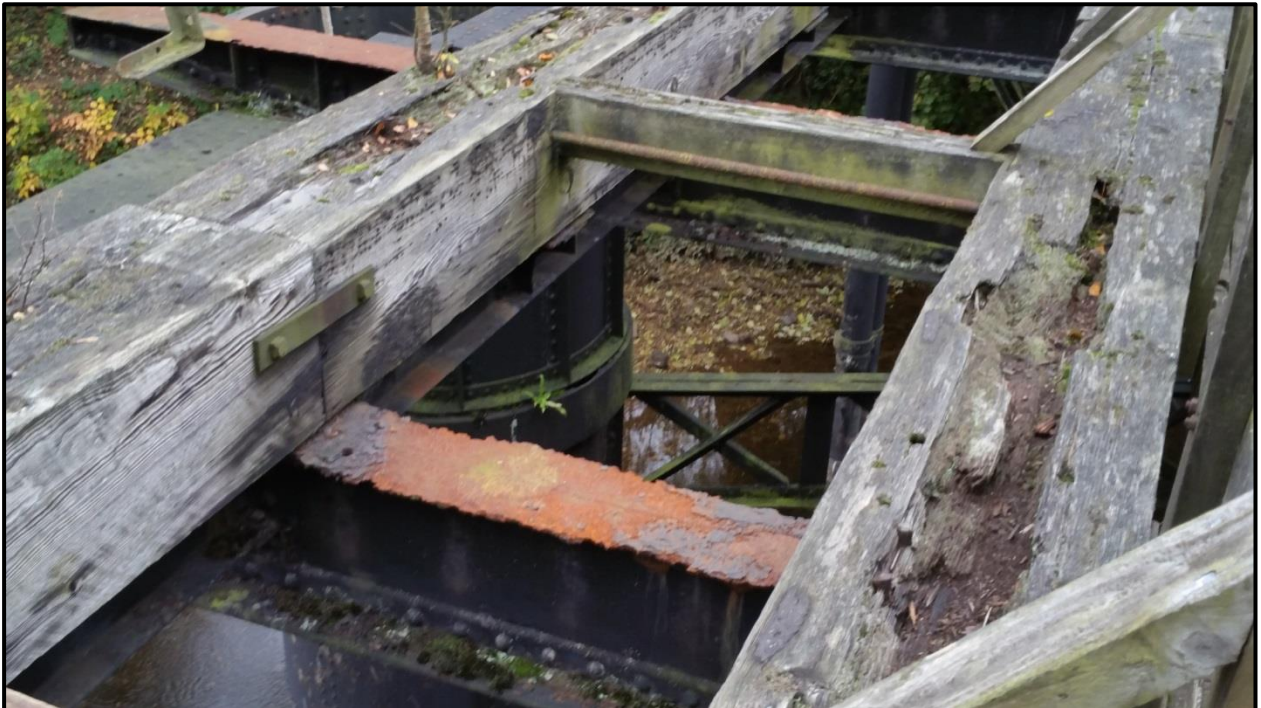
Picture 19. Transverse beam. Top flange
