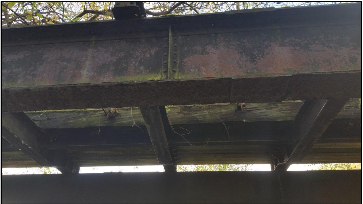
Picture 17. Jack rusting in main girders
