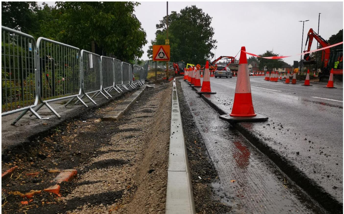
The footway/cycleway construction and kerb line installation on the A38 toward Gloucester from Cross Keys Roundabout is coming along well, with top-soil and surfacing to be started shortly.
