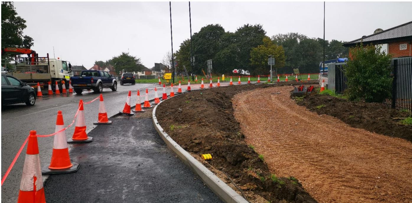
The footway/cycleway outside McDonalds has been constructed, ready for surfacing. We have also completed a gas main diversion.
