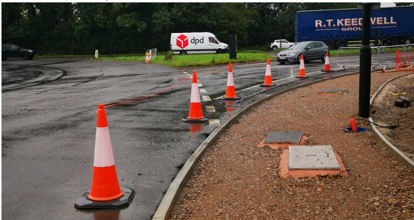
The kerbs are installed opposite the M&S verge for the new carriaway and cycleway/footway layout.
