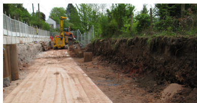
Installation of the piles
