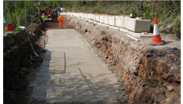
Completion of the Legato stabilisation blocks and construction of the concrete piling platform.
