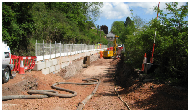
Handrail installation to ensure the separation of our workforce and piling operations.
