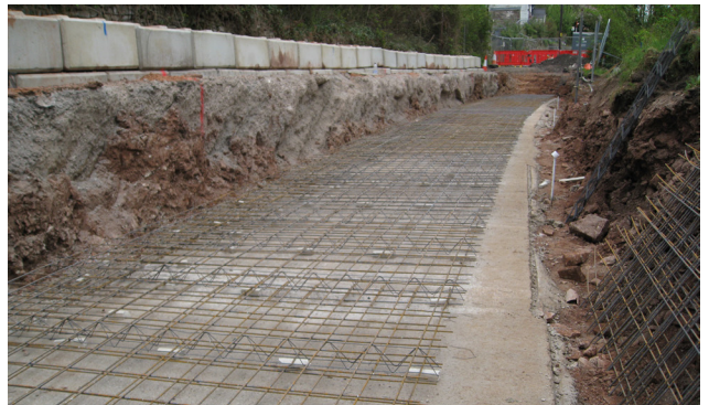
Construction of the concrete piling platform.
