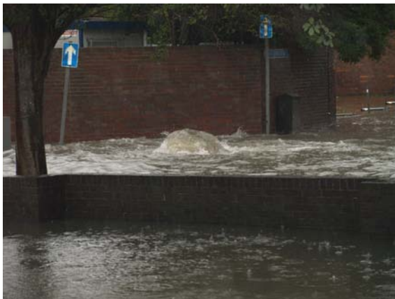
Burst manhole in Gloucester during the July 2007 floods.
