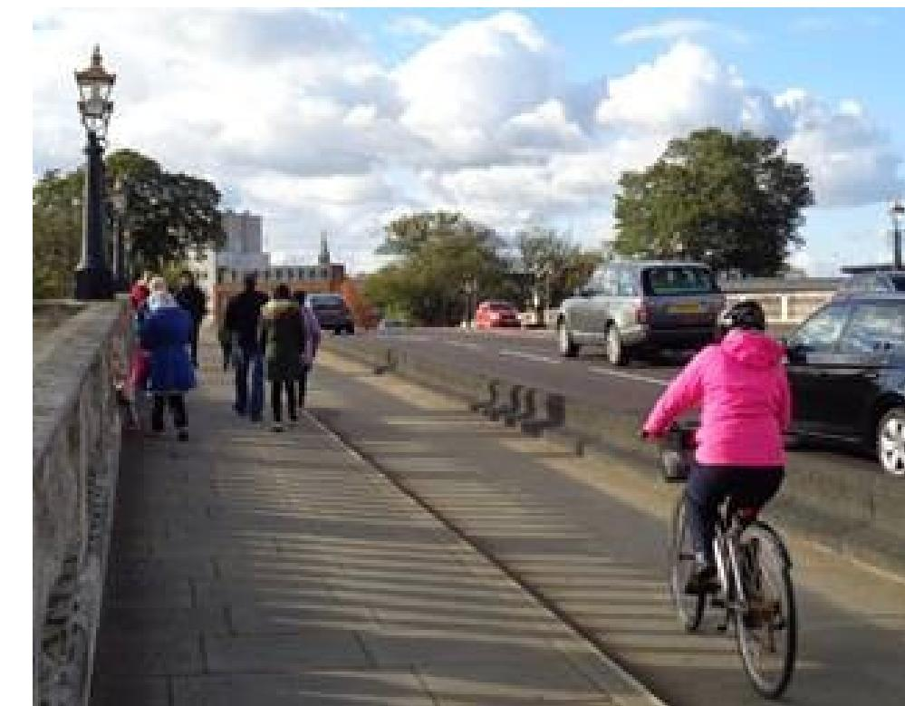
Typical cross-section east of Griffiths Avenue. Cycle track is at the same level as the road, below the footway.
