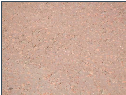
Photograph C.1.3 – Pigmented Hot Rolled Asphalt (Red binder + red coated chippings) (Preferred option)
