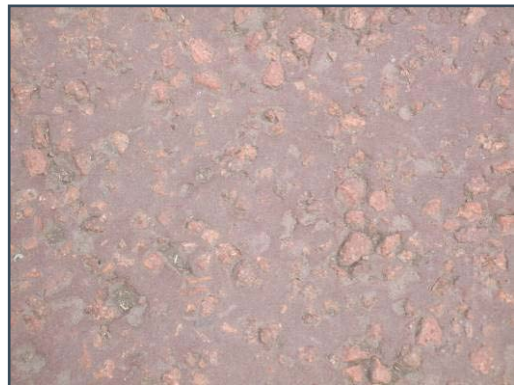
Photograph C.1.4 – Pigmented Hot Rolled Asphalt (Red binder + red coated chippings) (Coating removed to reveal decorative aggregate)
