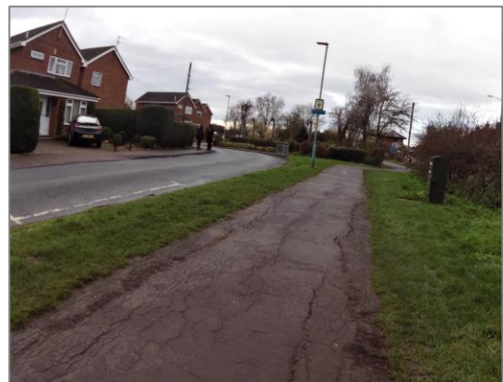
(d) Cracked surface of shared use path reduces effective width and limits cyclists speed, there are also two sharp bends in the distance (Knights Way).
