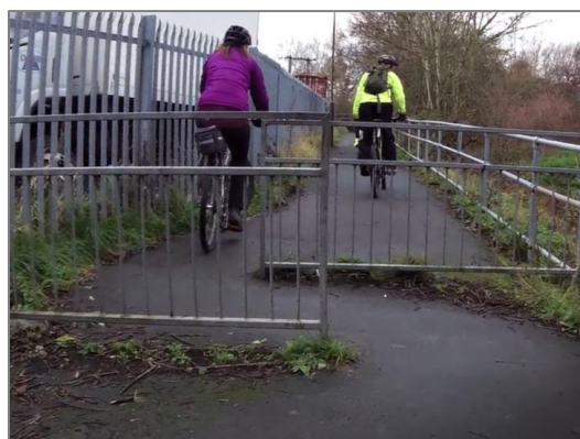
(n) Staggered barriers, such as these used on Route 13.2, should not be used and removed across the LCWIP network.
