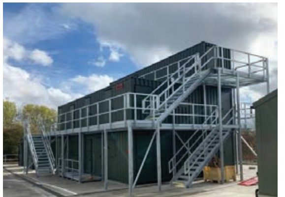
Example image of a Live Fire House
