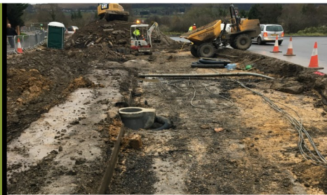
Installation of new drainage gullies
