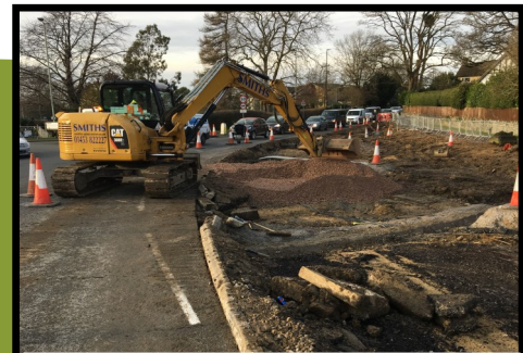
New stone to form road base layer
