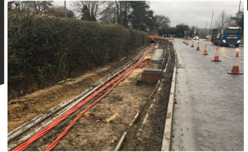
Western Power Distribution cables for diversion
