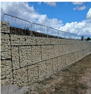
Photo 5: Gabion wall
