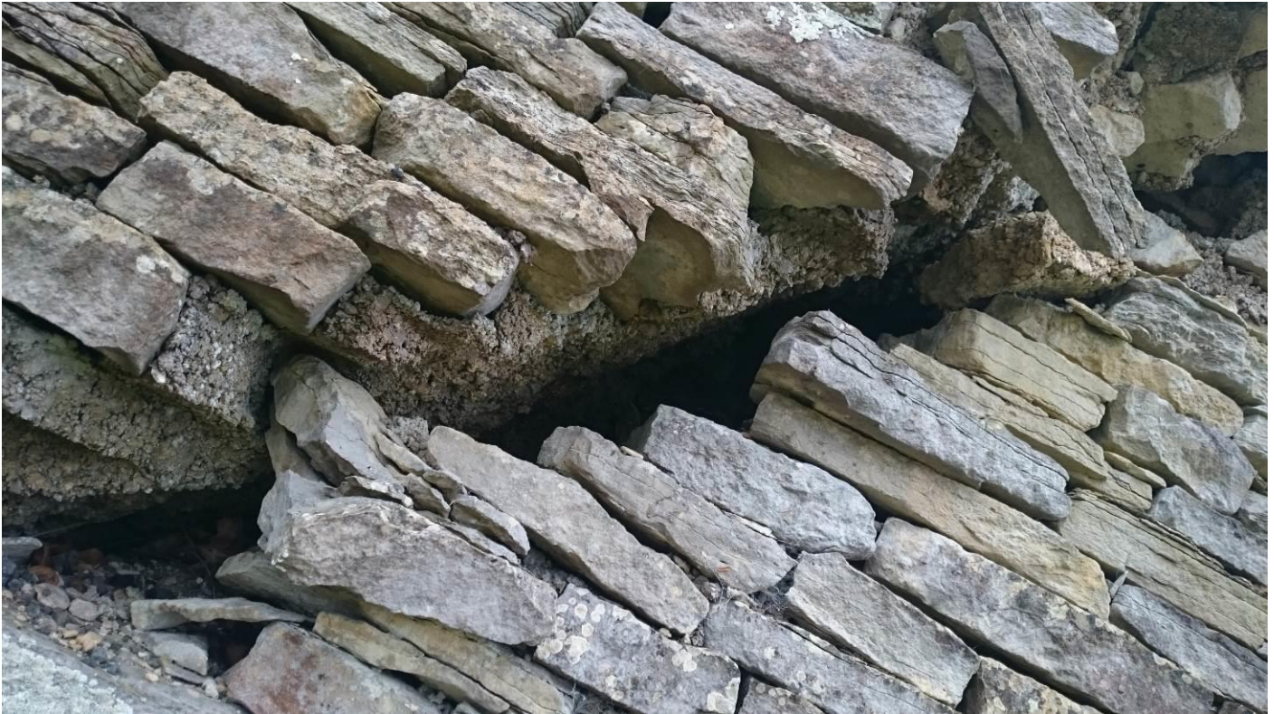
Photograph 5. Detailed of the retaining wall cracking and construction (25.11.2015)
