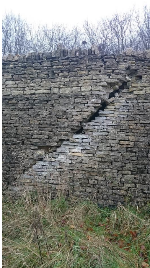
Photograph 3. View to the north of the retaining wall cracking and displacement (25.11.2015)
