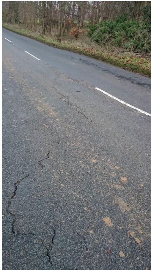
Photograph 10. Area 1 - View towards the east of the cracking within the eastbound carriageway (25.11.2015)
