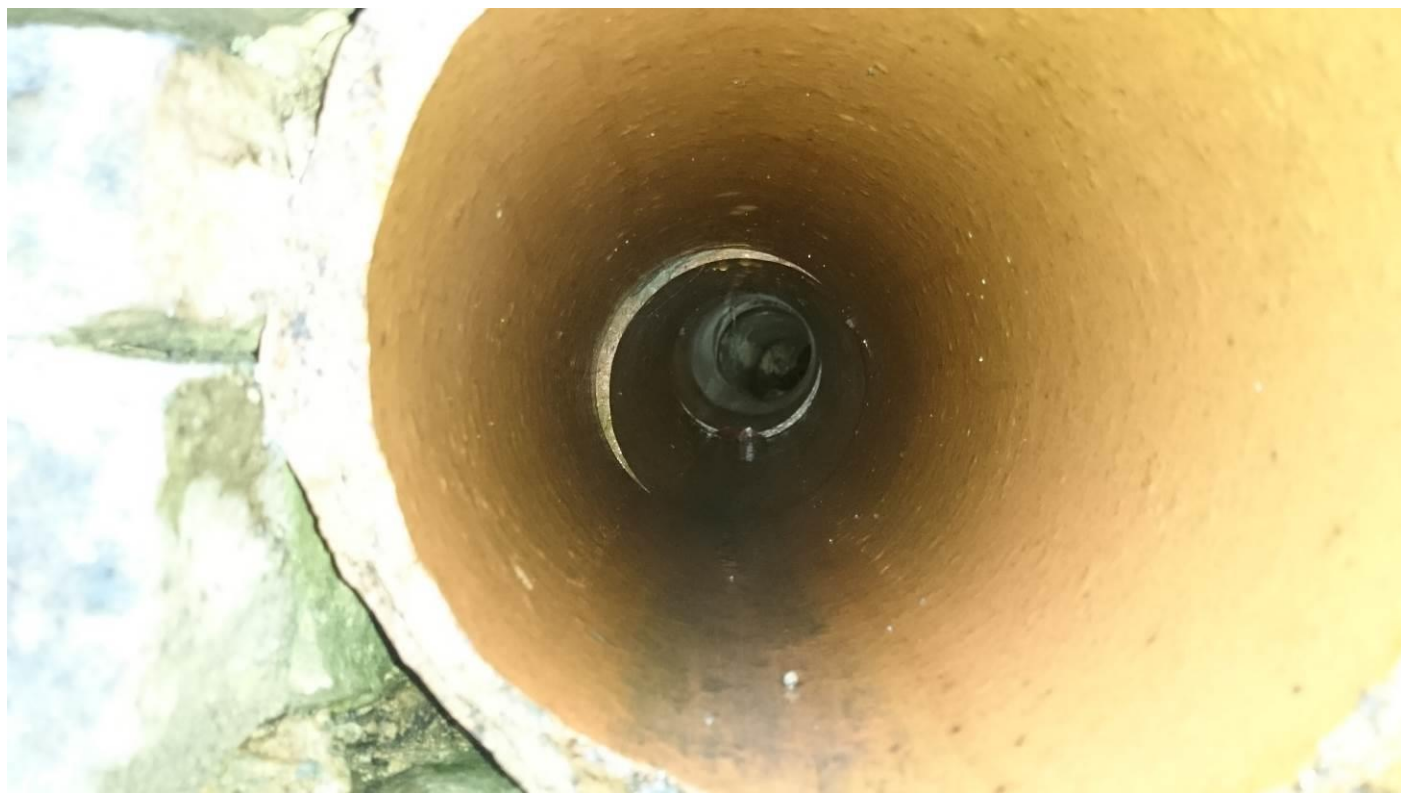
Photograph 7. Cracked drainage outfall pipe (25.11.2015)
