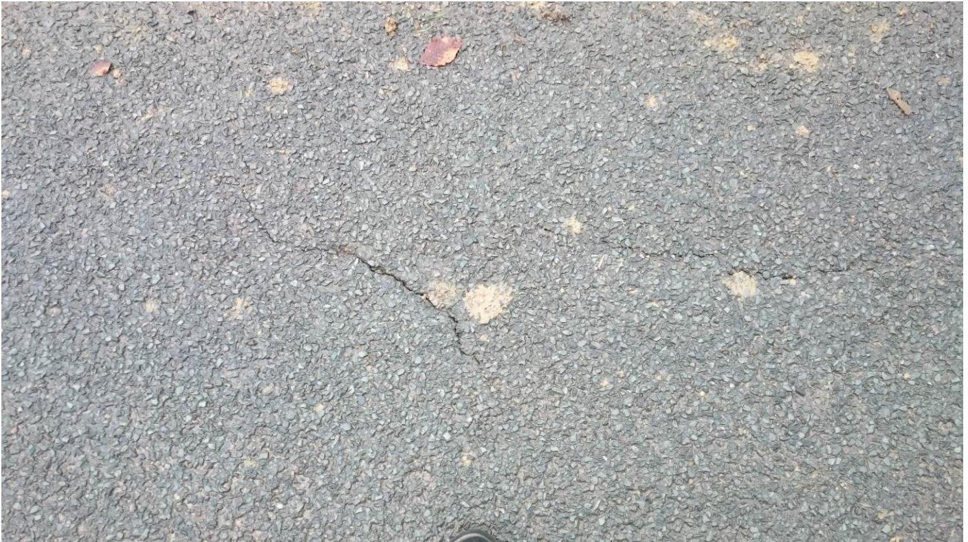
Photograph 13. Area 3 - Cracking within the eastbound carriageway (25.11.2015)
