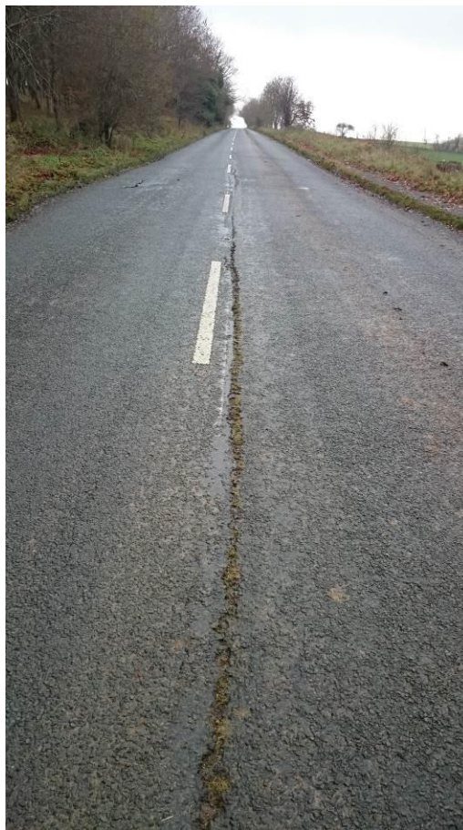
Photograph 12. Area 3 - View towards the west of the cracking along the centre of the carriageway (25.11.2015)
