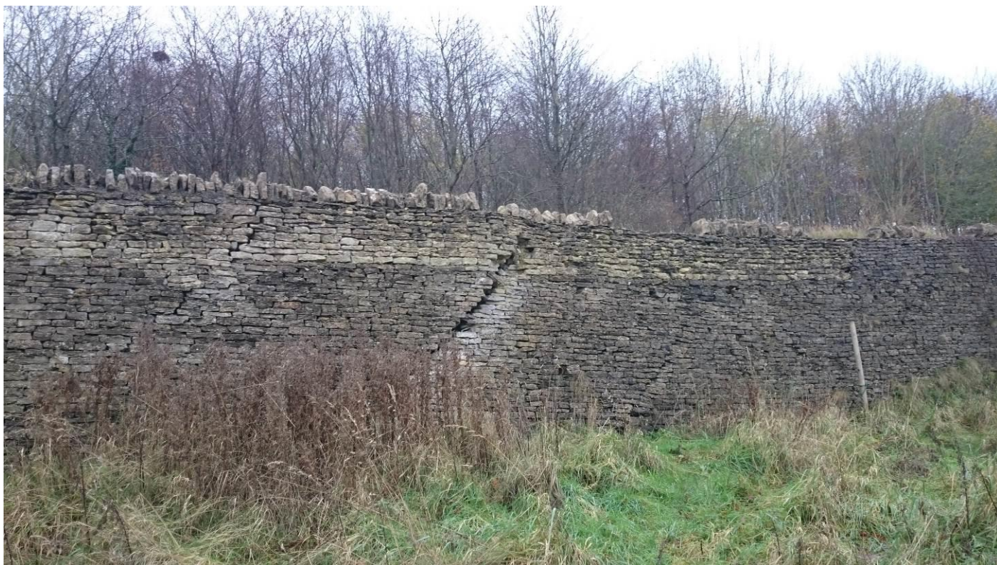
Photograph 1. View to the north of the retaining wall cracking (25.11.2015)
