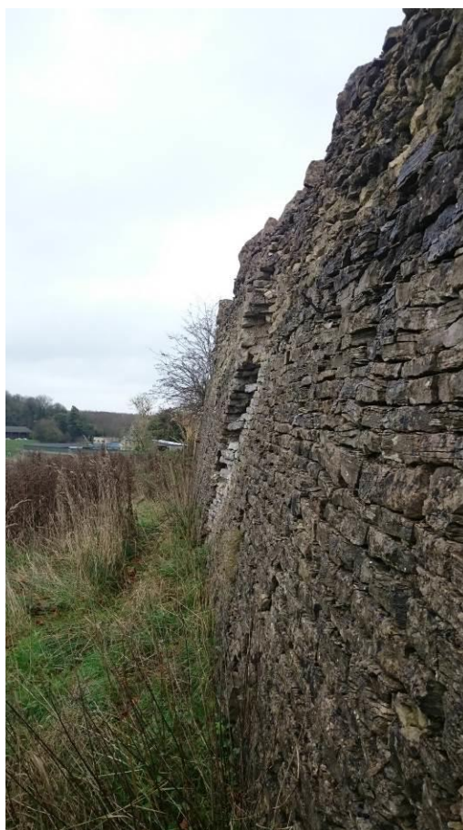
Photograph 4. View to the east of the retaining wall cracking and displacement (25.11.2015)
