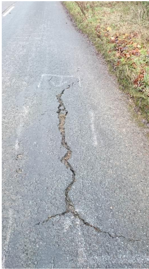
Photograph 9. Area 1 - Cracking within the westbound carriageway (25.11.2015)
