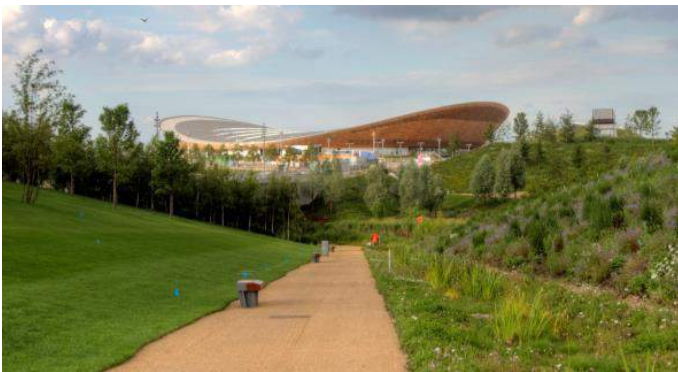
Figure 9-8 – Swale construction on the London 2012 Olympic Park (before and after)
