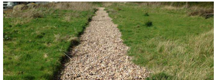
Figure 9-26 - Filter drain (SuDSwales)
