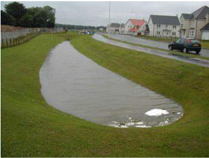
Figure 9-22 – Detention pond - full
