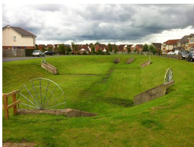
Figure 10-10 – Poor headwall design
