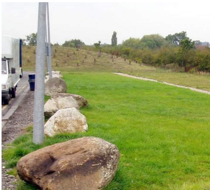
Figure 9-9 - Grass filter strip at the edge of a parking area (Susdrain)
