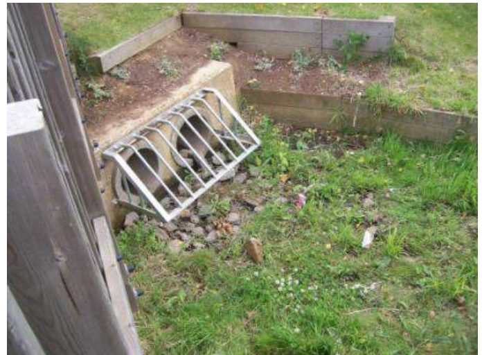
Figure 10-5 – SuDS outlet with trash screen
