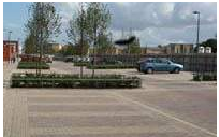
Figure 9-32 - Permeable pavement in a car park
