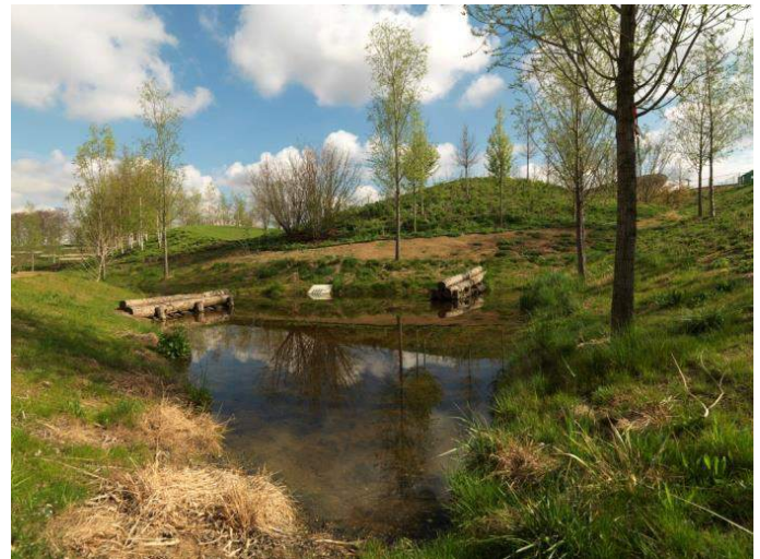
Figure 9-17 – SuDS pond showing inlet on far bank
