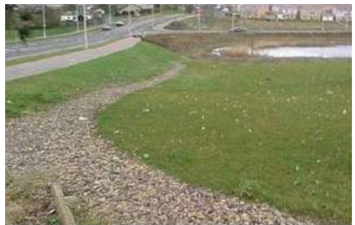
Figure 9-29 - Filter drain leading to pond
