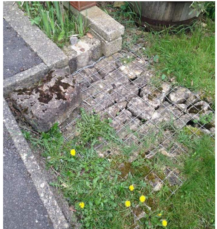
Figure 10-3 – Inlet and outlet using a stone basket
