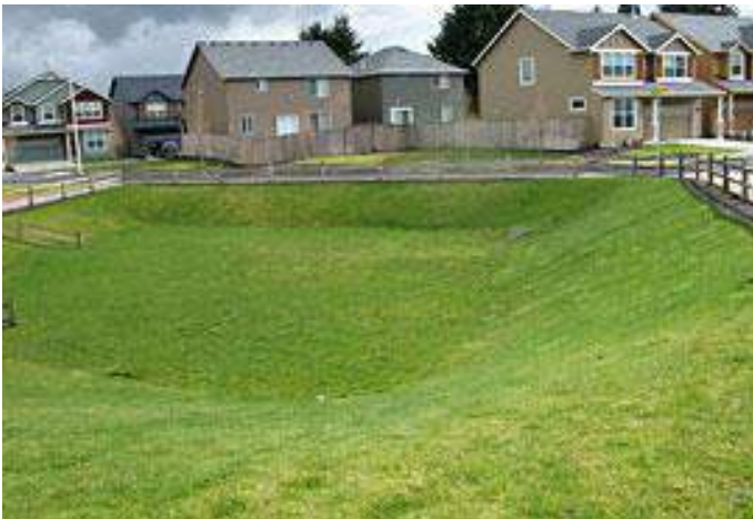
Figure 9-20 – Detention pond - empty
