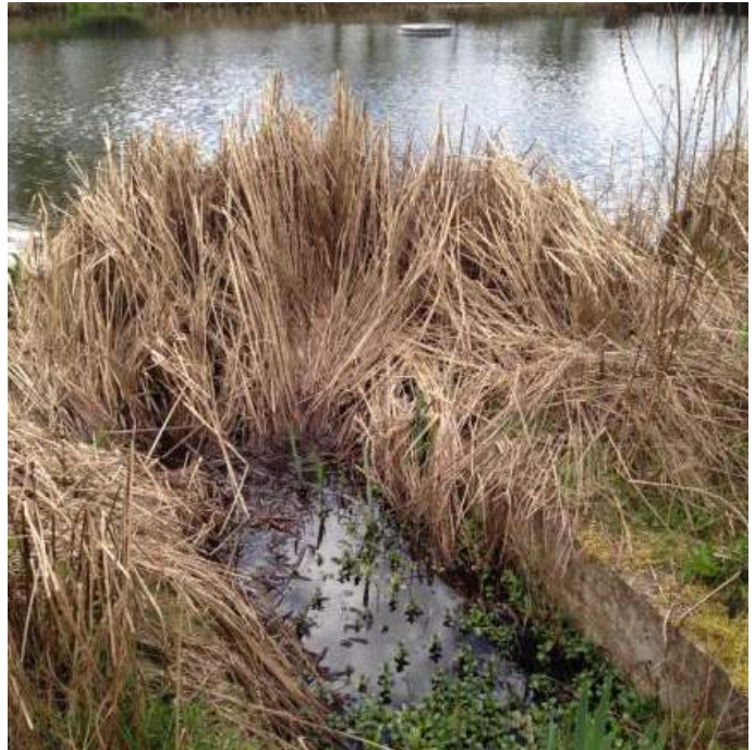
Figure 9-44 – Overgrown channel outfall
