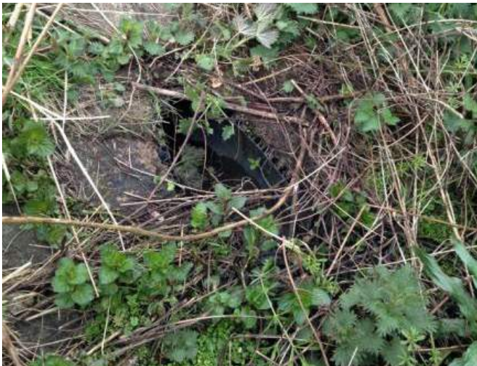
Figure 10-11 – Pipe inlet in need of maintenance
